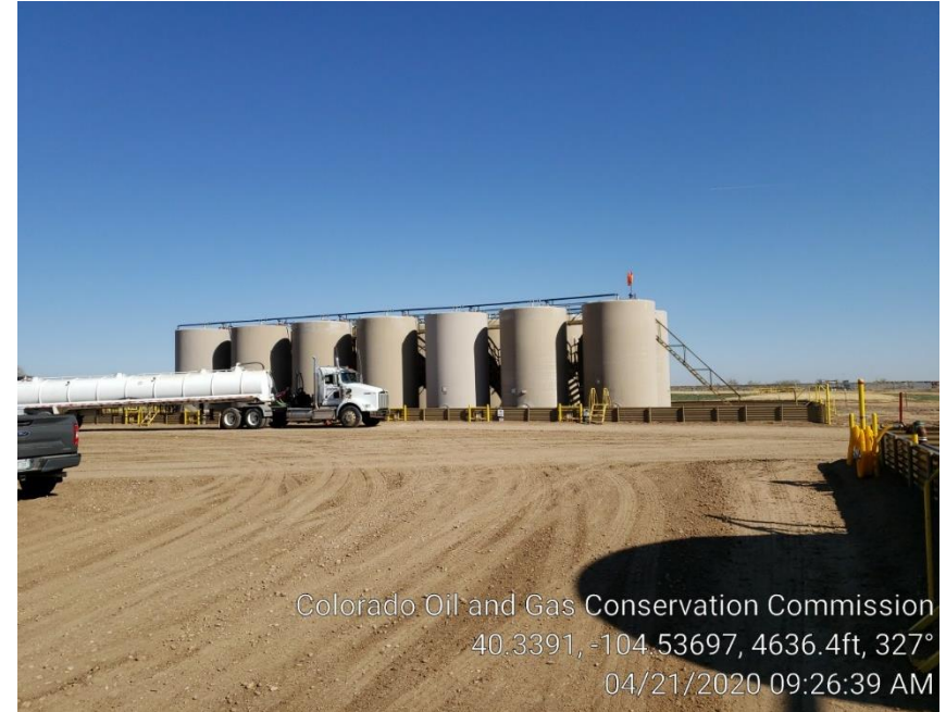
Photo #6 Produced Water Tanks
