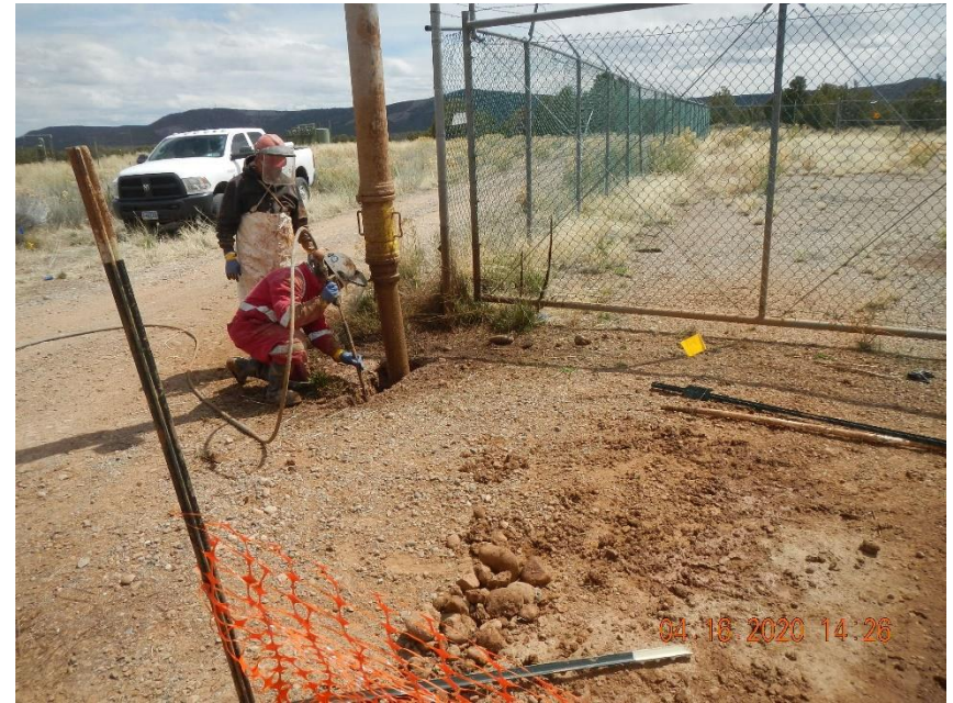
Hydro-vac crew potholing Catamount pipeline.
