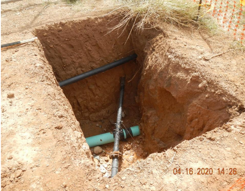
Excavated BP water gathering line, running top to bottom in this photo.
