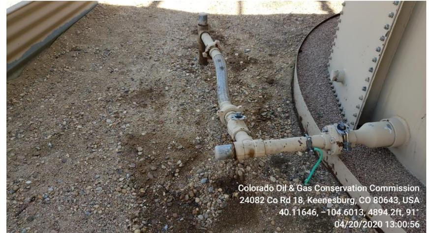
**Photo 13 Stained soil by fill line at tank battery.**
