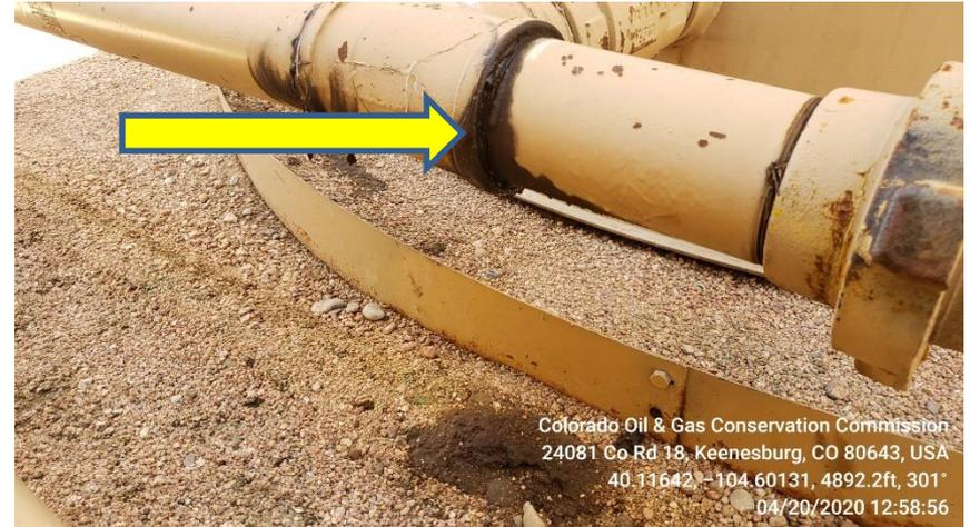
**Photo 15 Stained soil by fill line at tank battery.**
