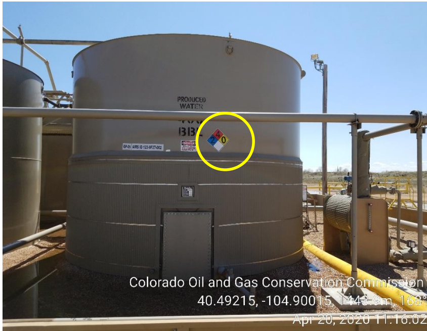
Photo 9: NFPA placard installed
