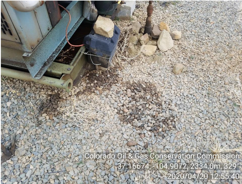
PHOTO 3: AREA OF IMPACTED SOIL NEAR ENGINE SKID. Conduct maintenance on equipment, cleanup stained material and review self inspection processes. CA DATE 4-25-20.
