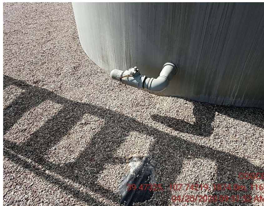
staining is gone
