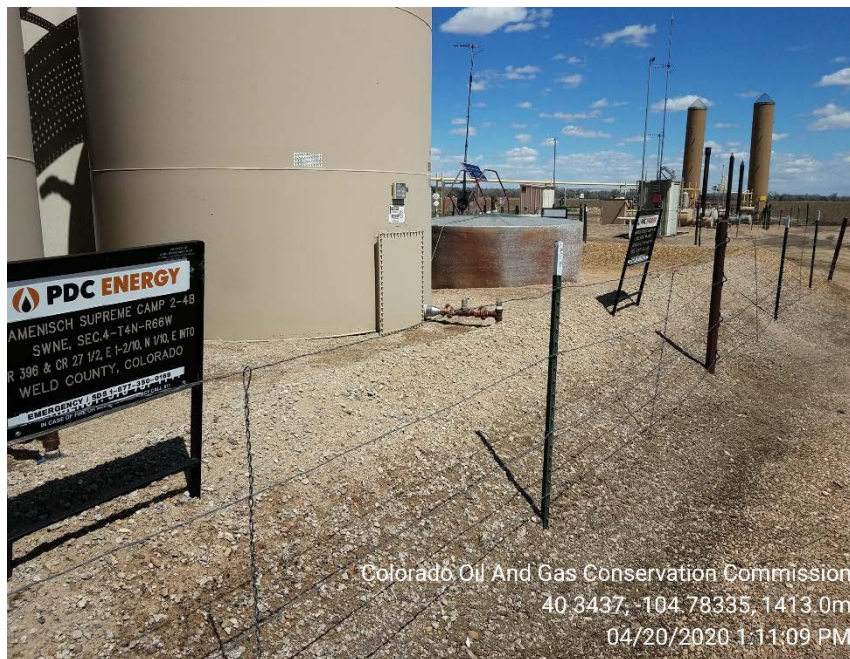
Crude oil tank berm
