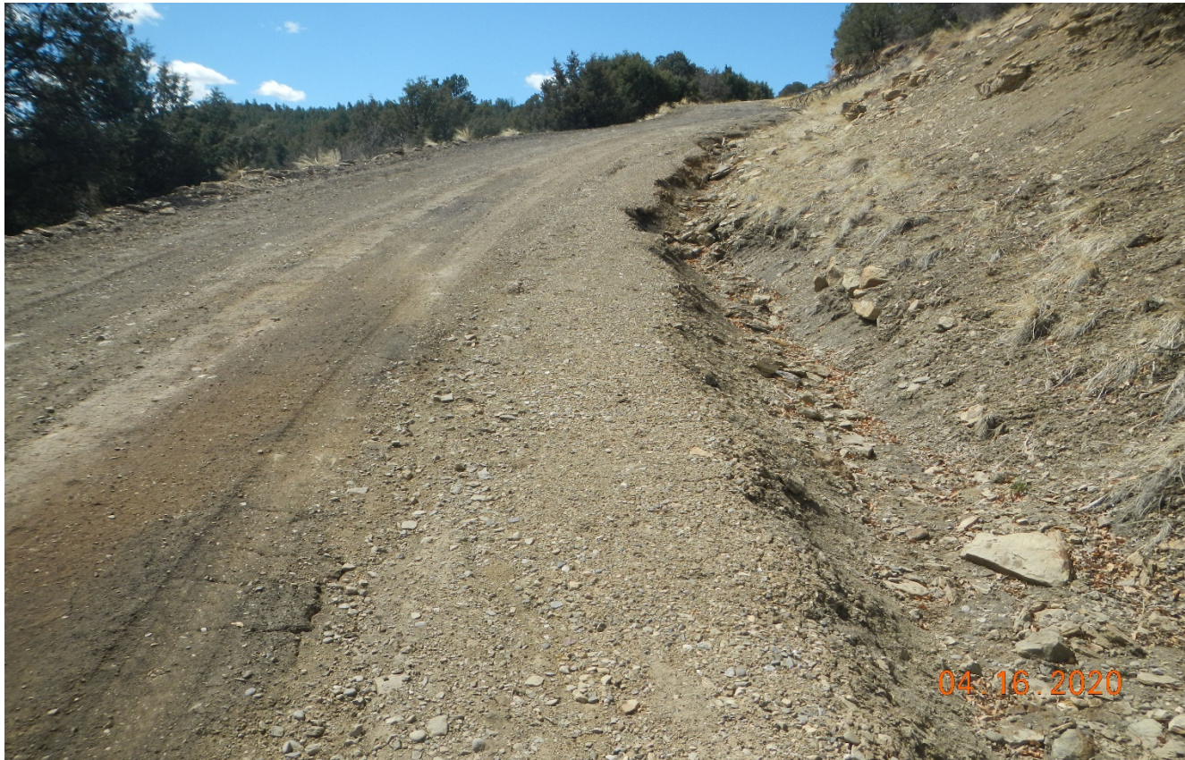
Photo 2. There is erosion occurring along the main road ascending the hill to the location.
