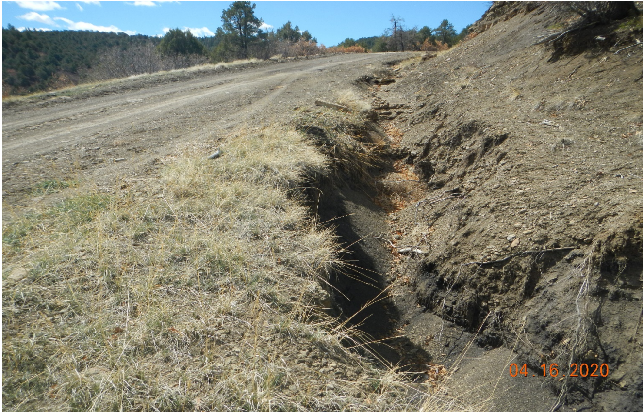
Photo 1. There is an erosion gully that has form along the main road at Lat/Long:37.081525,-104.69693.
