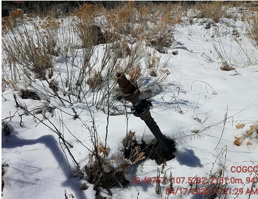
Unmarked flow lines
