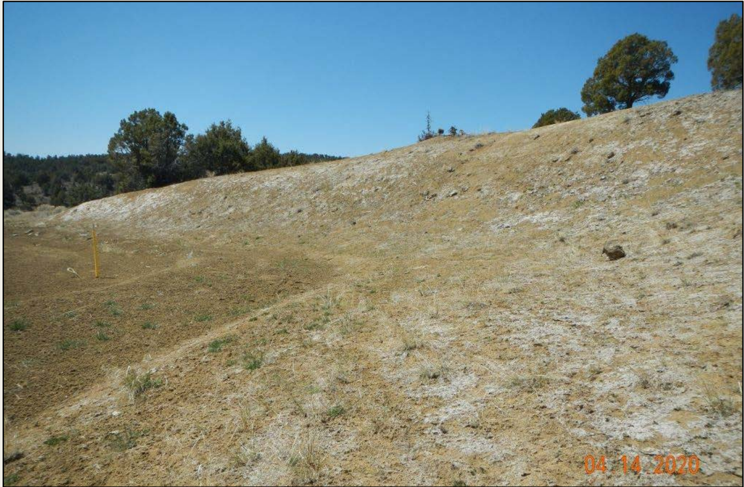
Photo 2. View of the northwestern project area facing southward. Cut-slopes appear to be re-seeded, hydromulch remains on slope.
