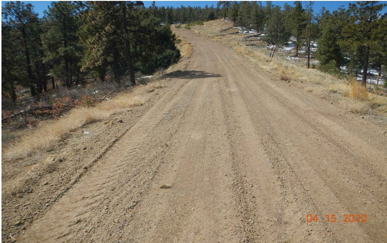
Photo 5. The road has been regraded where erosion was observed.
