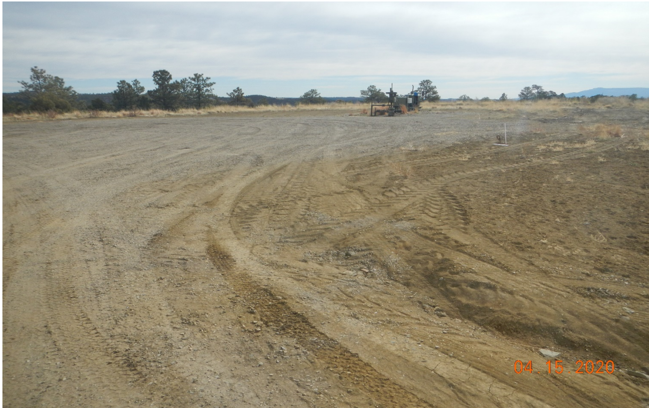
Photo 6. Facing east toward the well site.
