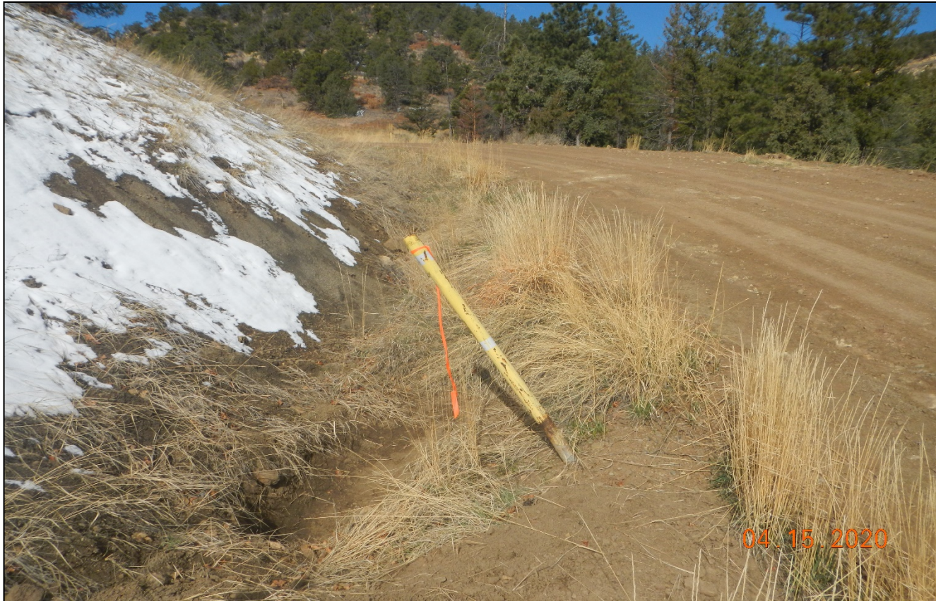
Photo 1. The culvert along the main lease road has been maintained.
