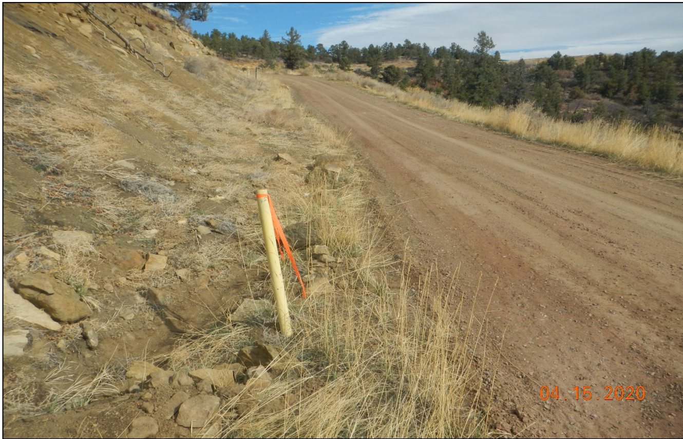
Photo 3. The culvert along the main lease road has been maintained.
