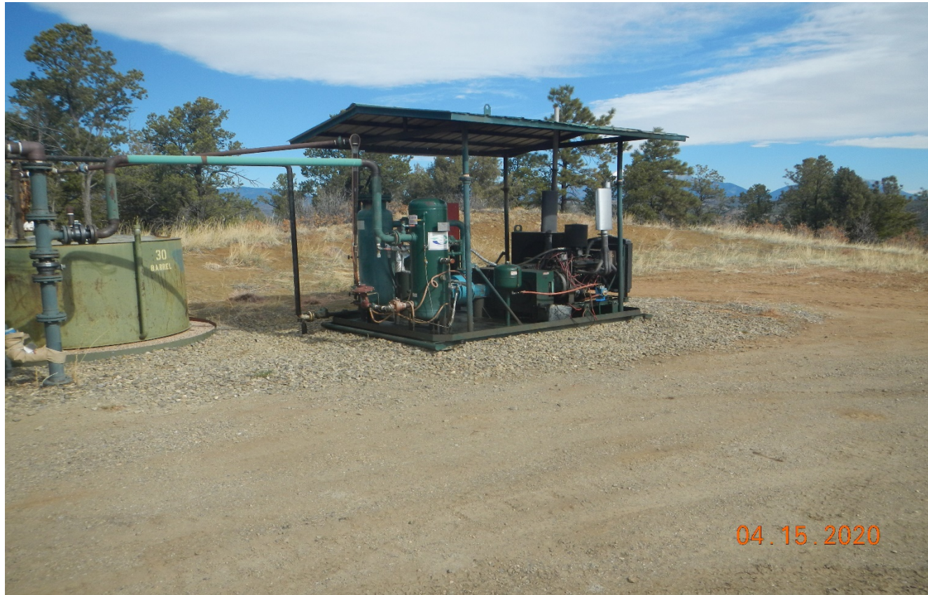
Photo 5. The exhaust pipe which was laying on the ground has been removed.
