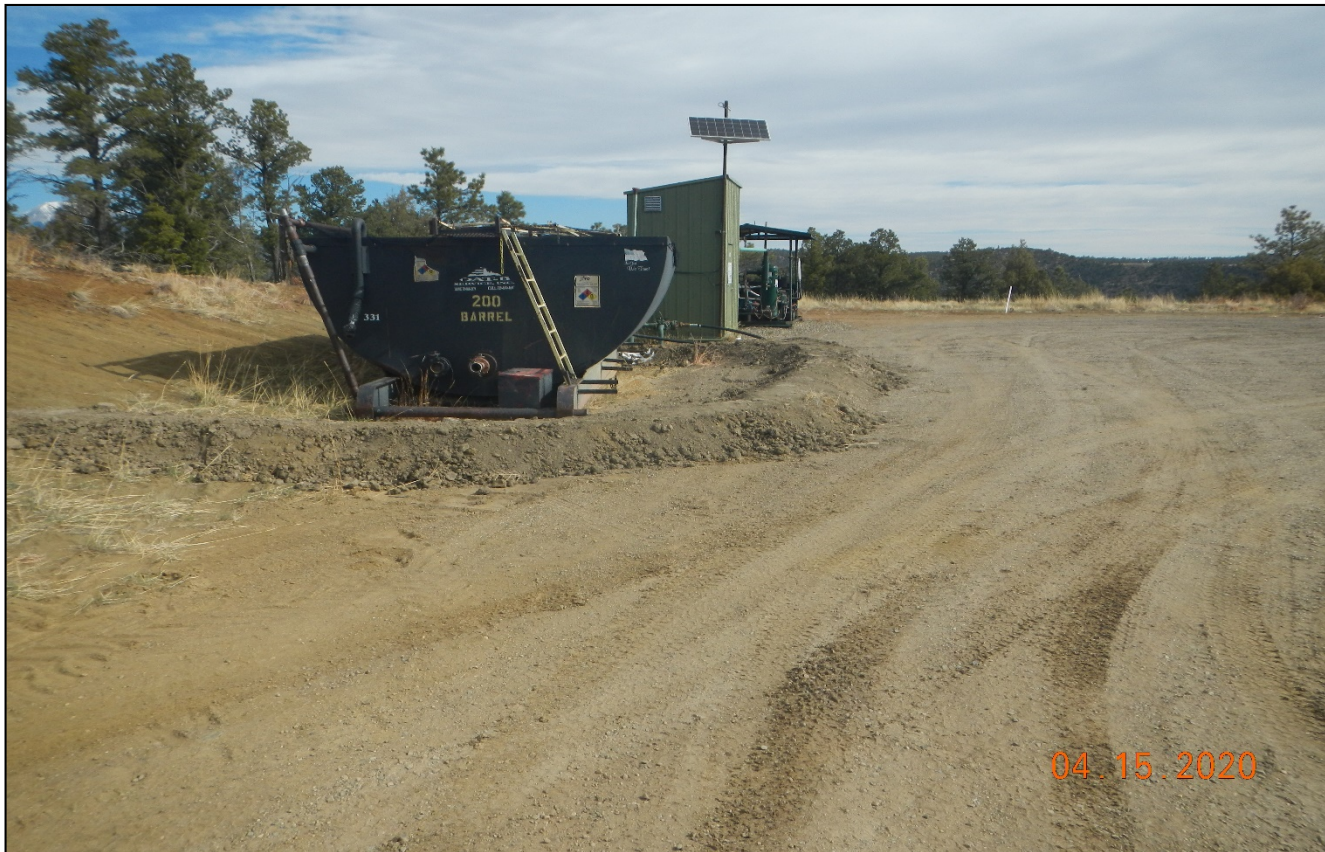
Photo 4. A berm has been installed around the open topped tank.
