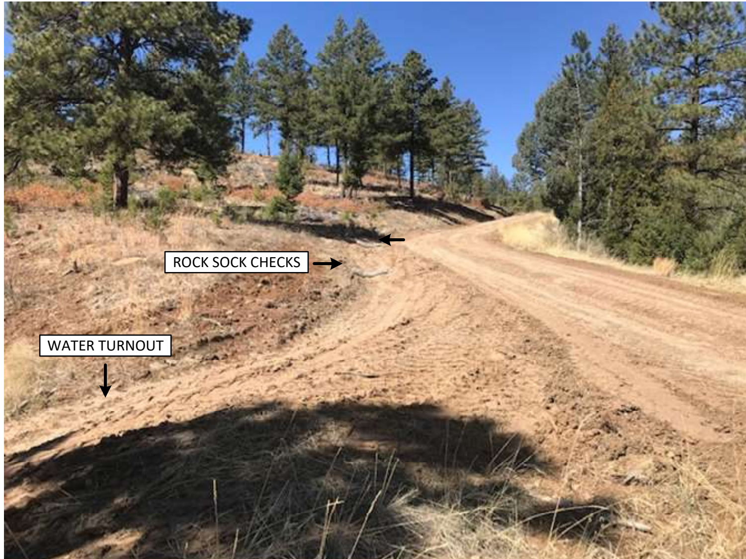
PHOTO 1: THE ACCESS ROAD TO LOCATION WAS SURFACE CROWNED TO ESTABLISH SHEET FLOW AND ELIMINATE THE TIRE RUTS. A WATER TURNOUT WAS INSTALLED TO DIVERT RUN OFF AWAY FROM THE ACCESS ROAD TO UNDISTURBED NATURAL VEGETATION. ROCK SOCK CHECKS WERE PLACED IN THE DITCH LINE FOR SEDIMENT CONTROL.
