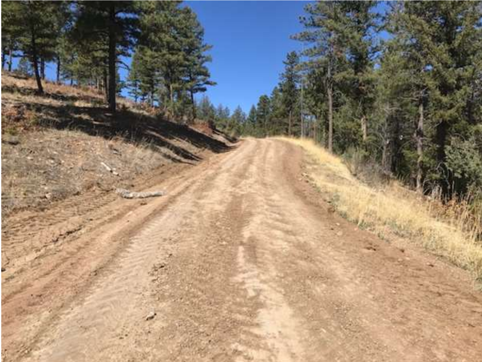
PHOTO 2: THE ACCESS ROAD TO LOCATION WAS SURFACE CROWNED TO ESTABLISH SHEET FLOW AND ELIMINATE THE TIRE RUTS. ROCK SOCK CHECKS WERE PLACED IN THE DITCH LINE FOR SEDIMENT CONTROL.
