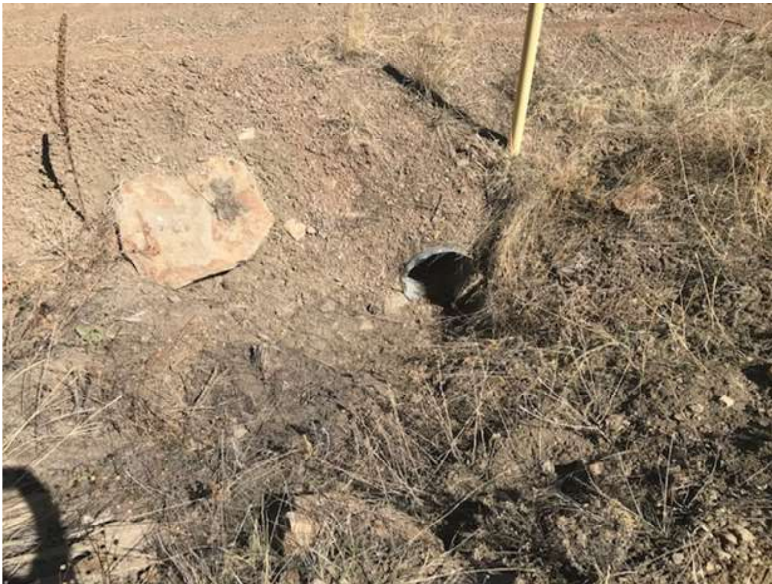
PHOTO 3: THE SEDIMENT ACCUMULATION WAS REMOVED FROM THE CULVERT INLET ALONG THE ACCESS ROAD.
