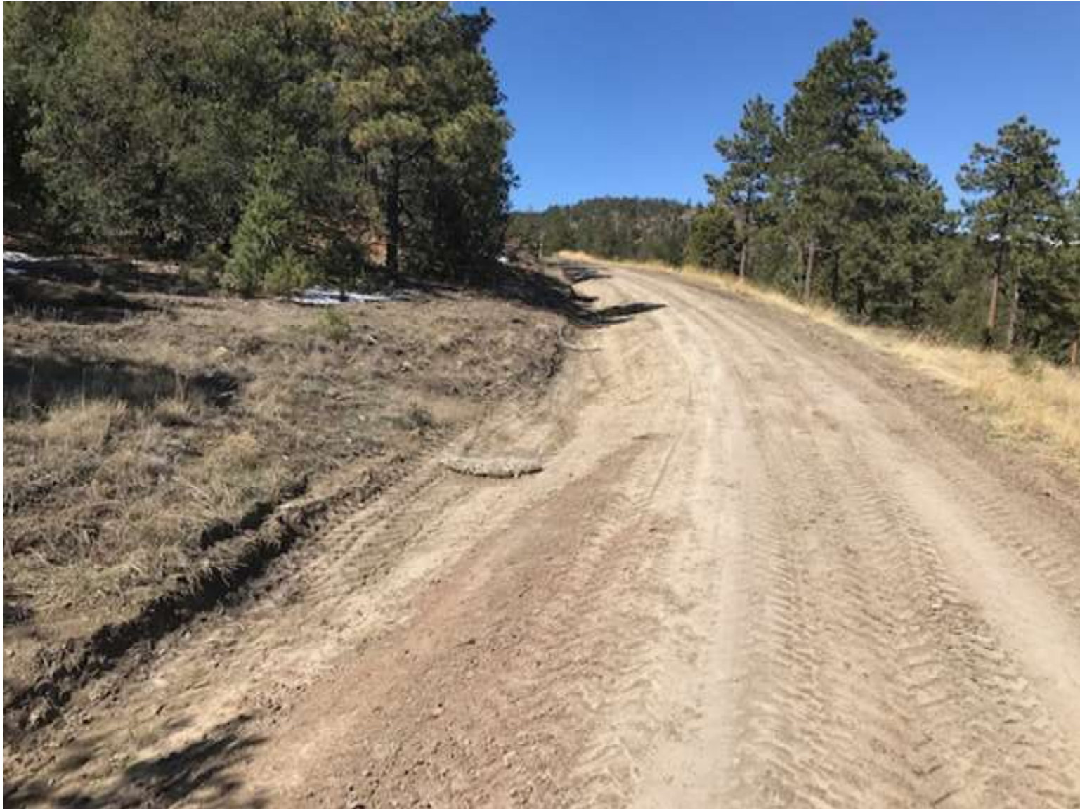
PHOTO 4: THE BAR DITCH WAS BACK FILLED AND THE SOIL WAS COMPACTED WITH THE BACK HOE TIRE TO ELIMINATED THE DITCH CUTTING ALONG THE MAIN ROAD. ROCK SOCK CHECKS WERE PLACED IN THE DITCH LINE FOR SEDIMENT CONTROL.
