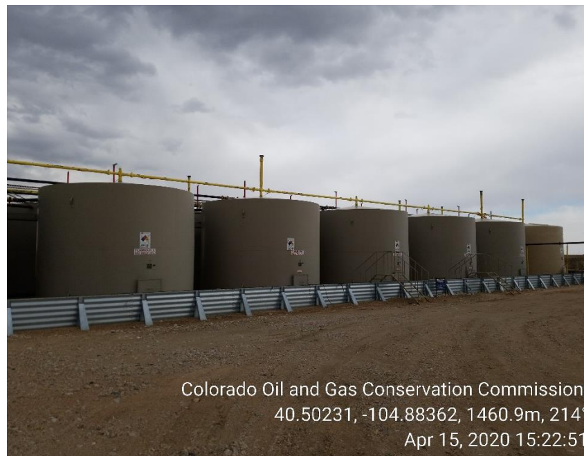
Photo 2: Tank Battery
