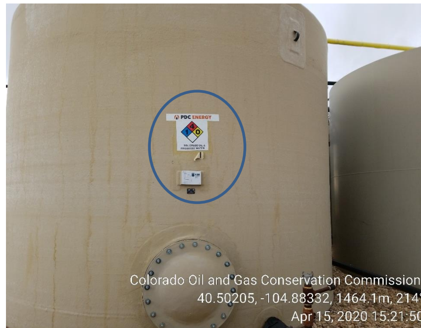
Photo 4: No BBLs installed
