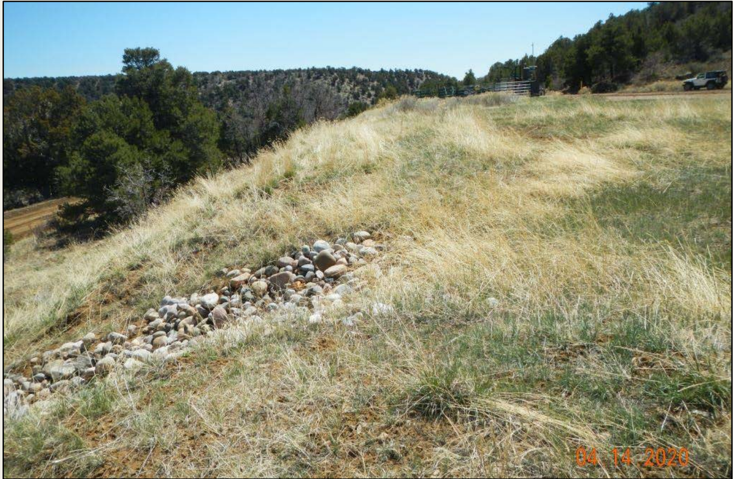
Photo 2. View of the northeastern fill slope from the northern corner facing southeastward. Revegetation is progressing, largely with western wheatgrass and sand dropseed.
