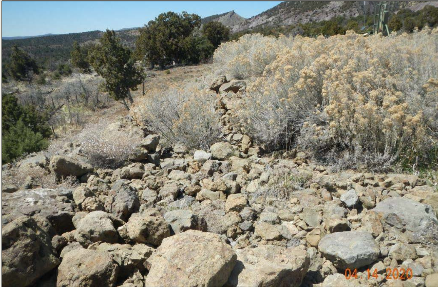
Photo 2. View of the southern fill slope from the southern corner facing westward. Revegetation is with rubber rabbitbrush and western wheatgrass. Interim reclamation area, is largely rock fill.
