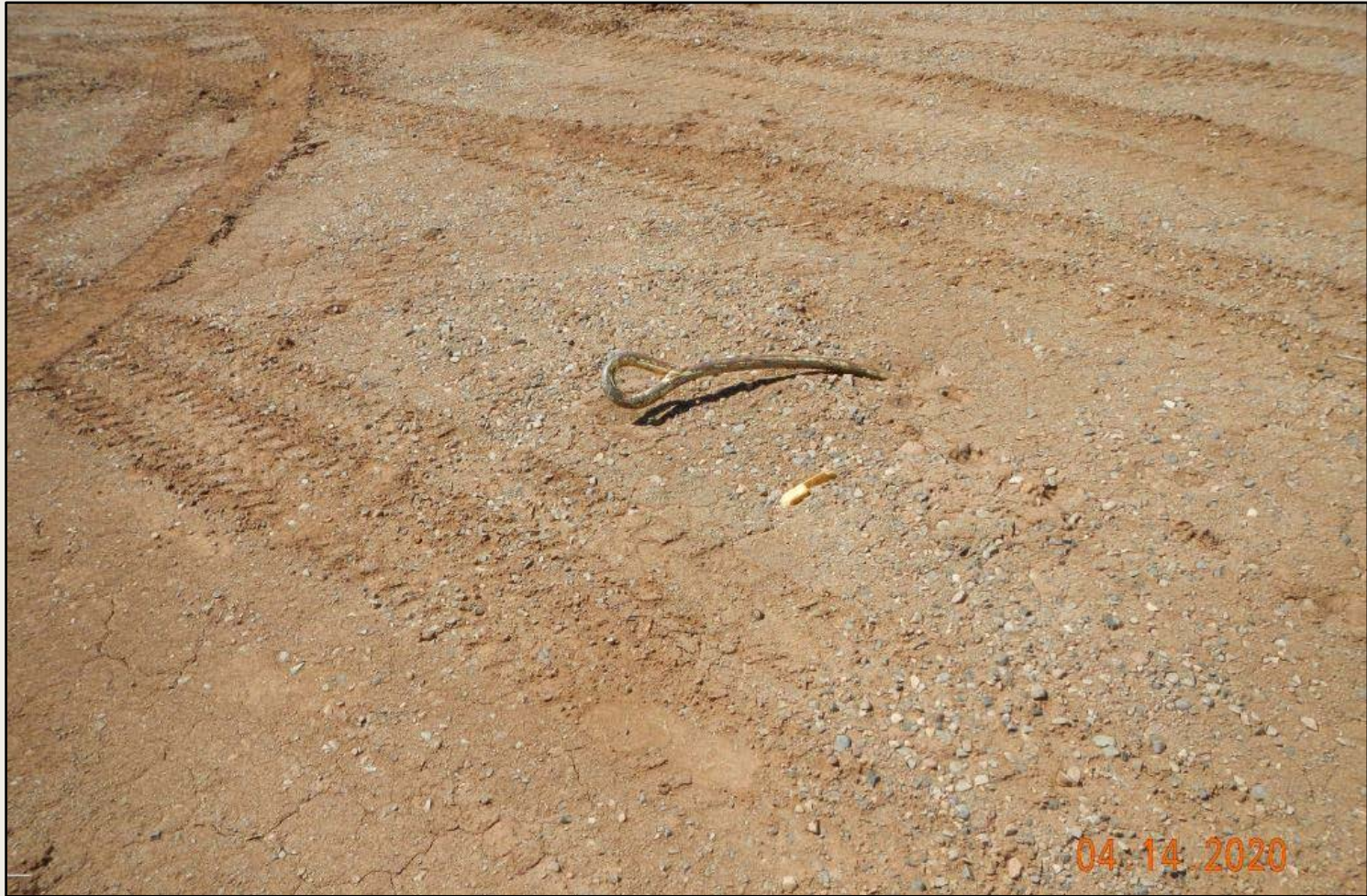
Photo 4. View of unmarked rig anchor on the well pad.
