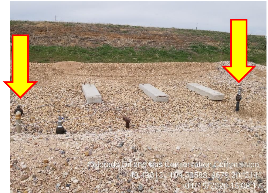
Photo 4 – Unmarked Risers at NE Berm
