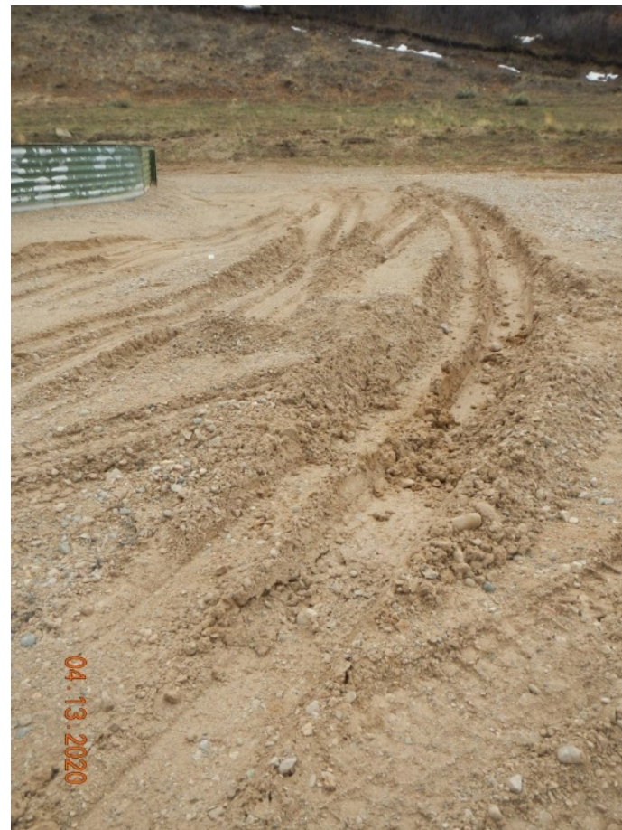
Photo#5: Rutting on Pad on Southwest corner
