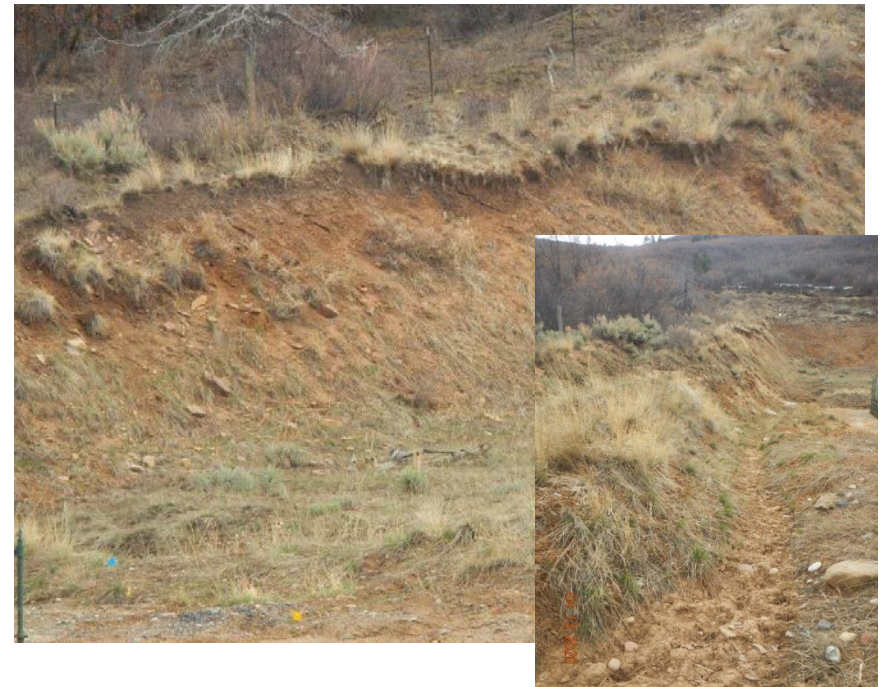
Photo#7: Cut slope and soil migration.
