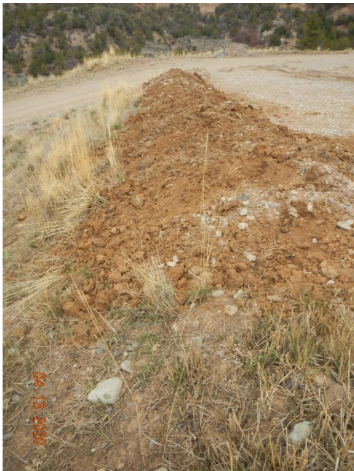
Photo#4: Loose soil with no down gradient BMP.
