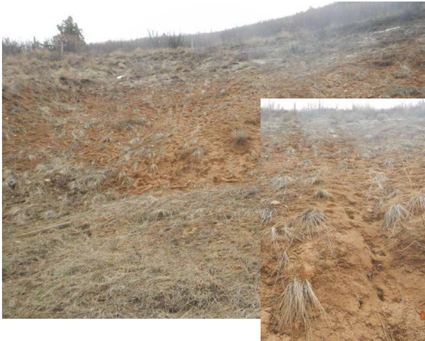
Photo#6: Cut slope; initiating erosion.
