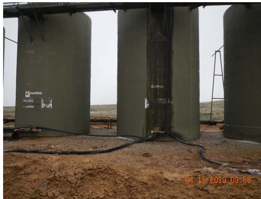
Photo 3. Missing or incomplete tank labels.
