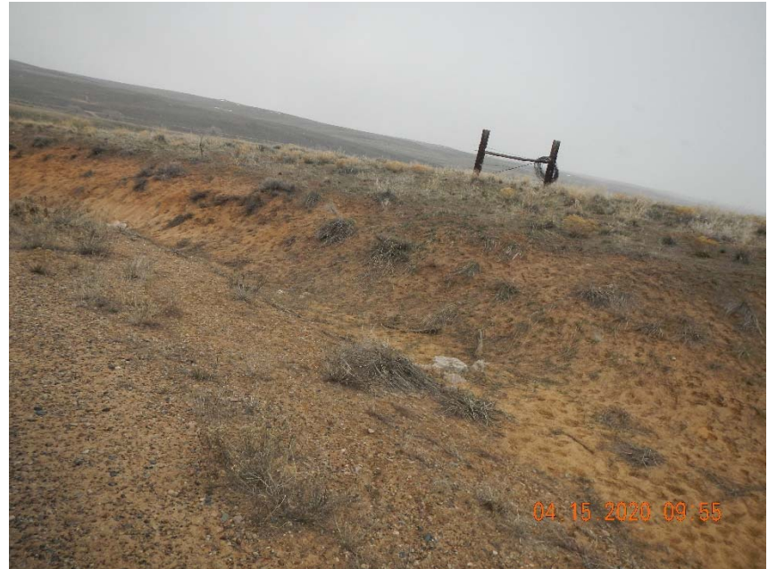
Photo 5. Sediment transport down access road ditch. Photo taken from same spot as photo 4 but looking down access road ditch away from location.
