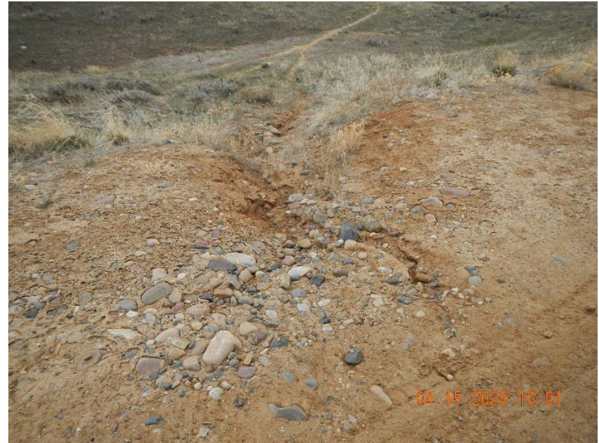
Photo 7. Example of rill leaving access road.
