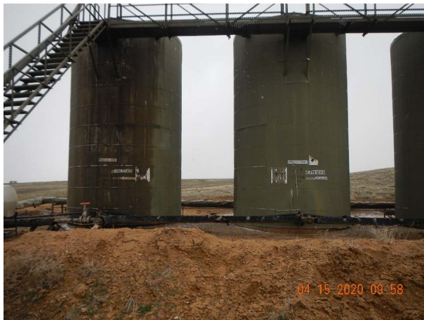
Photo 2. Missing or incomplete tank labels.
