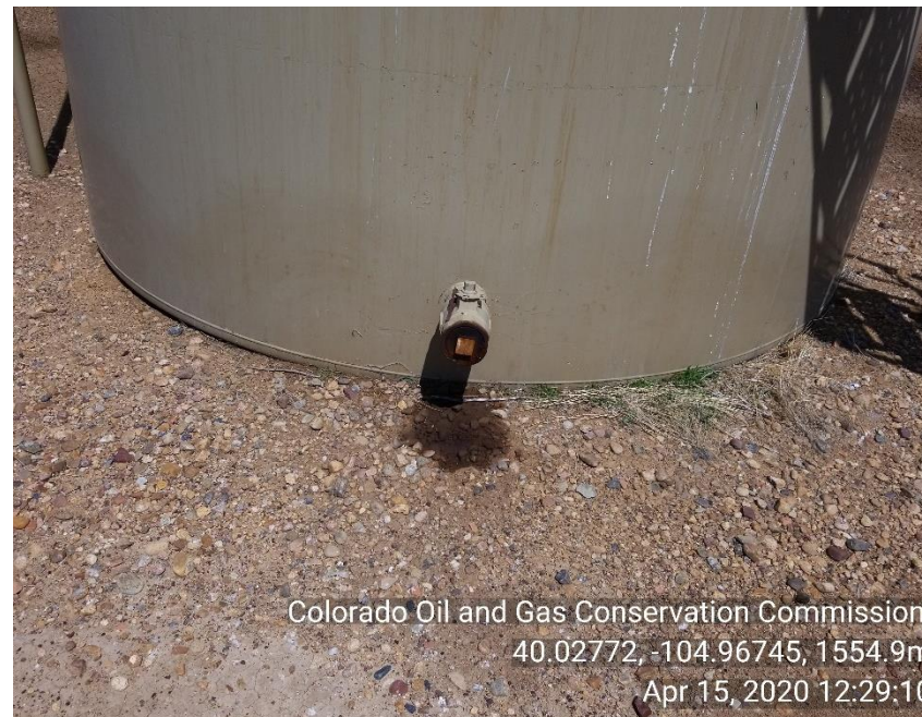
Photo 4 Mechanical issue and stained soil crude oil tank load line.
