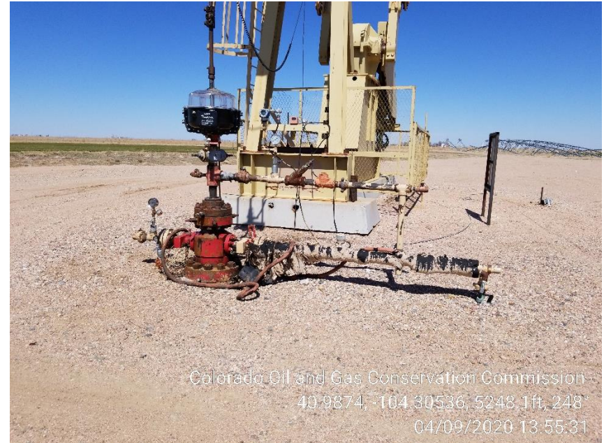
Photo 2 – Wellhead, Stained Soil removed
