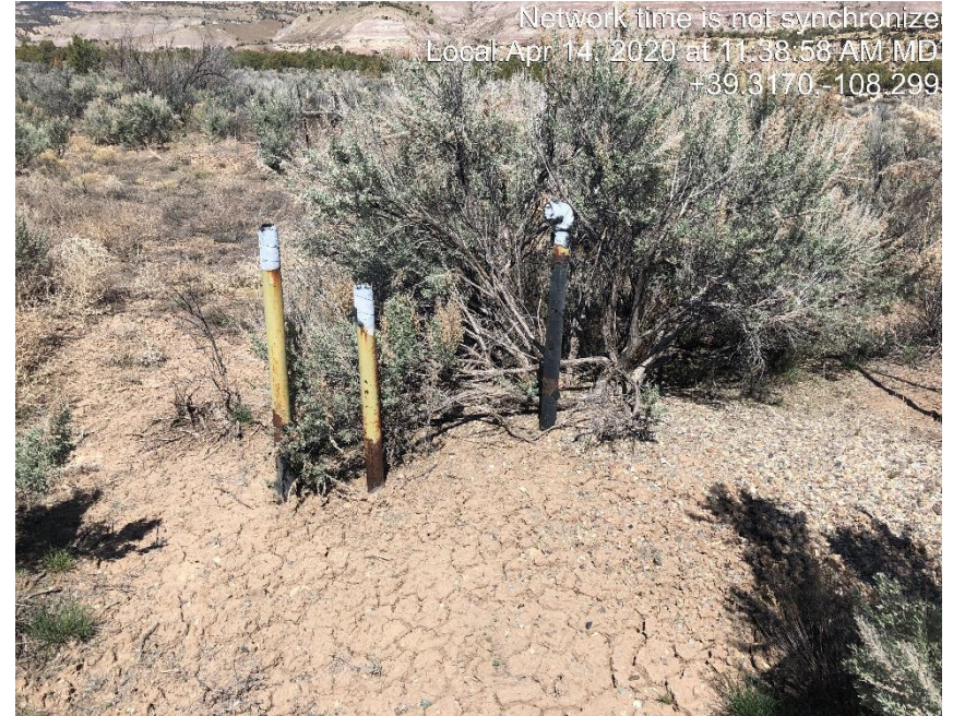
Photo #0964 Multiple flowline risers not LO/TO.
