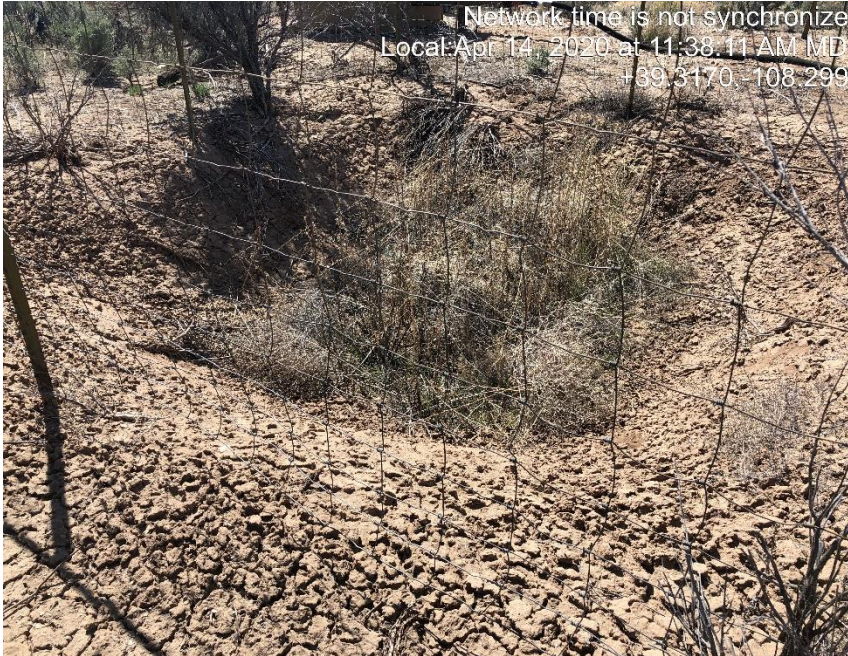
Photo #0963 Debris inside both pits. No netting on pits.
