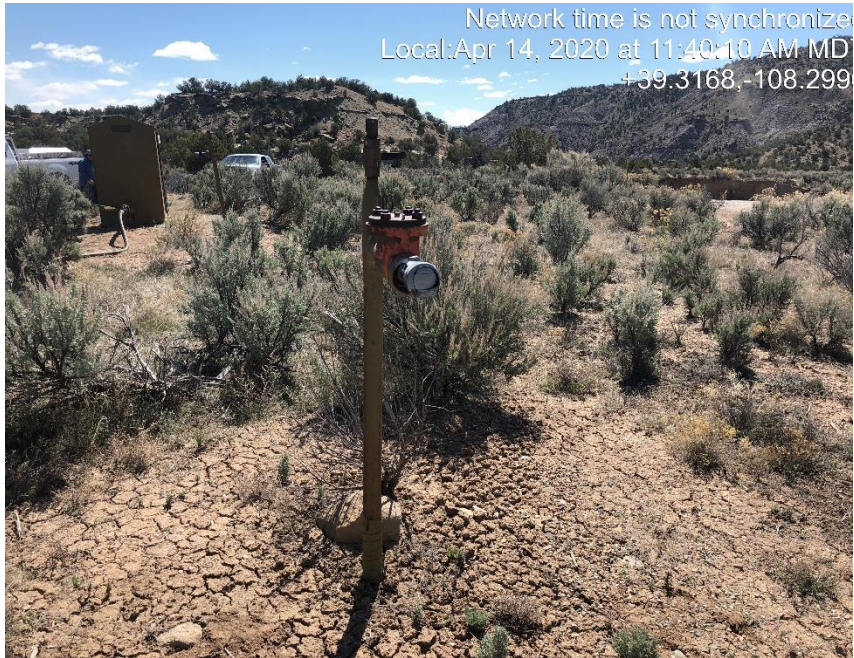
Photo #0965 Multiple flowline risers not LO/TO.
