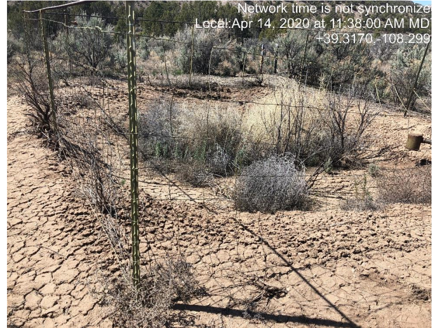
Photo #0962 Debris inside both pits. No netting on pits.
