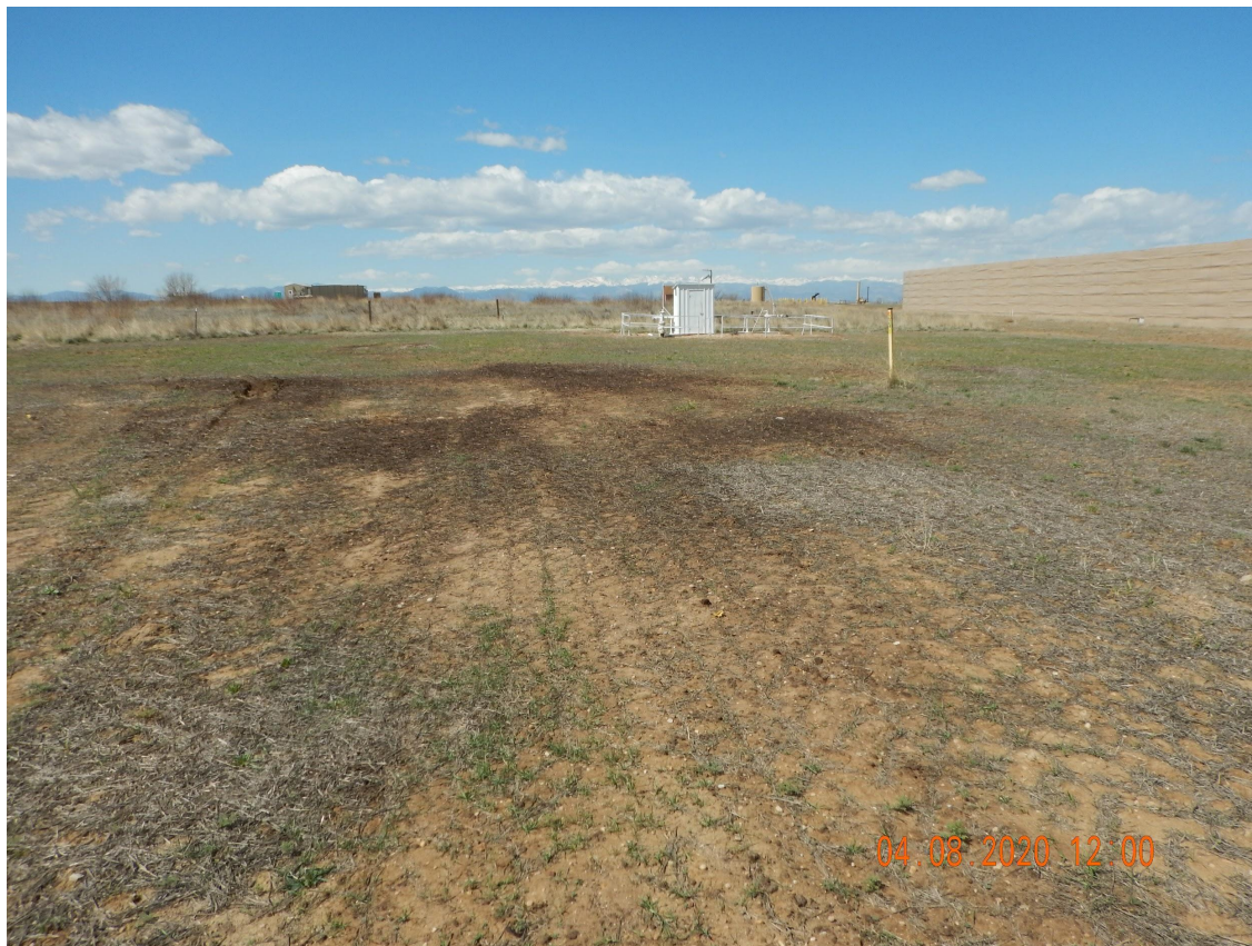
Photo 5. Photo taken from the associated offsite tank battery location, facing West. Photo illustrates Operator has performed final reclamation activities with the evidence of drill rows and germination. However, not all equipment has been removed.
