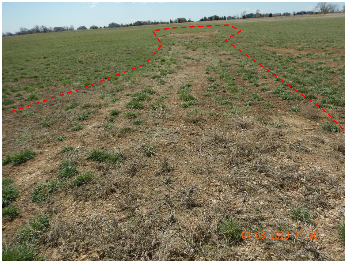
Photo 1. Photo taken from the well location entrance, facing South. Photo illustrates Operator has failed to remove all gravel and perform reclamation per Rule 1004 standards.
