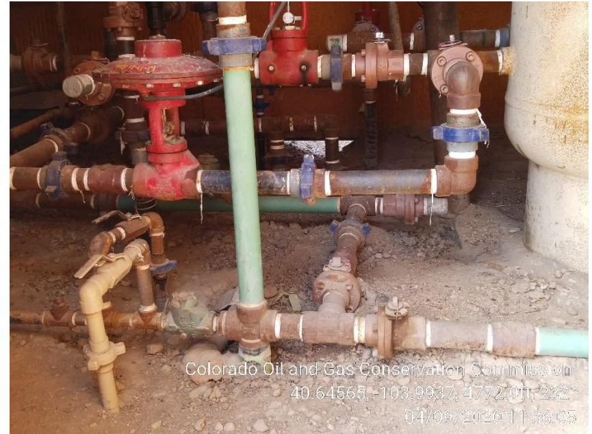
Photo 4 – Cleaned Soil in Heater Treater Shed
