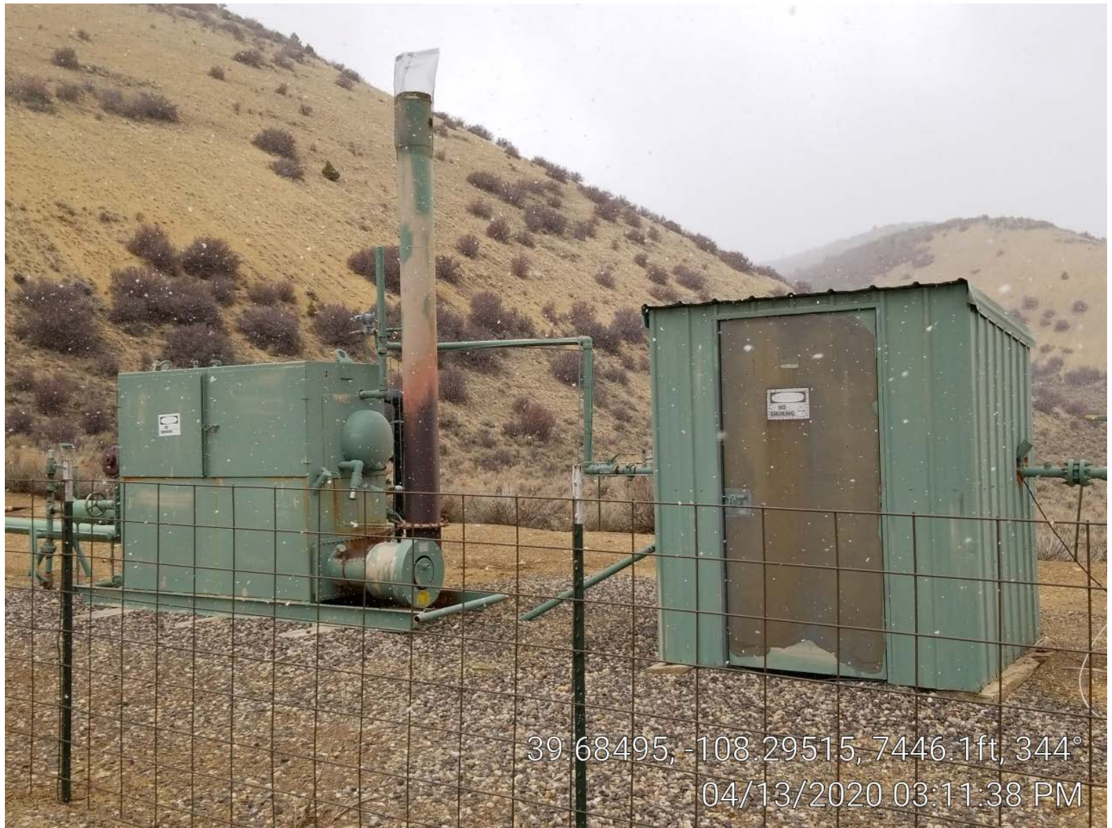
Photo 4. Separator & meter building.
