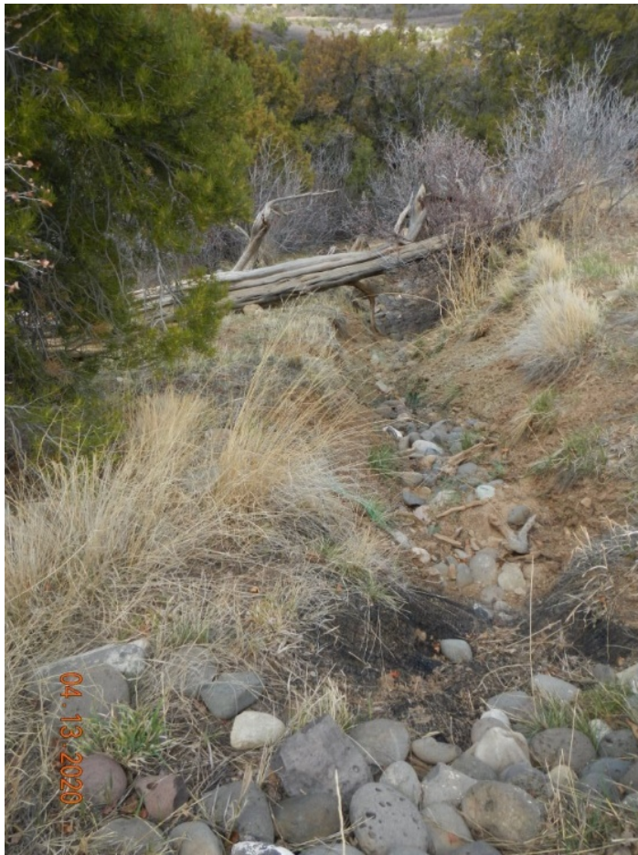
Photo#6: BMP at base of Fill.
