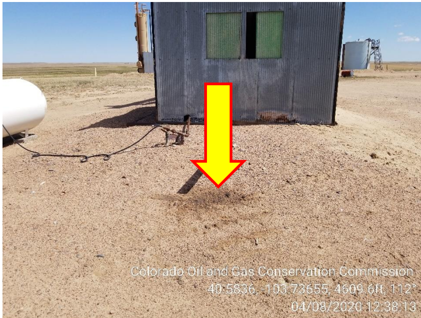
Photo 9 – Stained Soil at Exhaust
