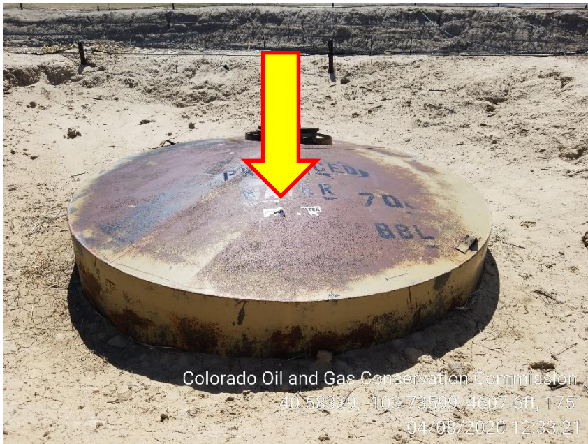
Photo 5 – Produced Water Tank NFPA label has faded
