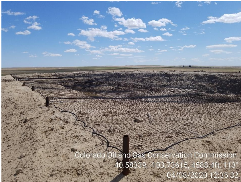
Photo 3 – Pit, Wildlife Netting has been installed
