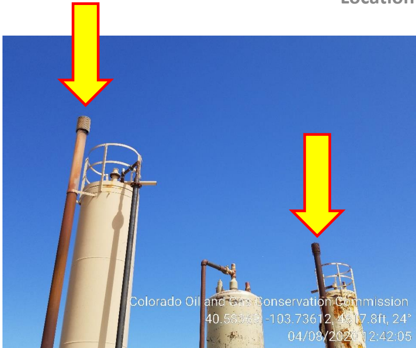
Photo 13 – Wildlife Screens have been installed to Heater Treater Stacks
