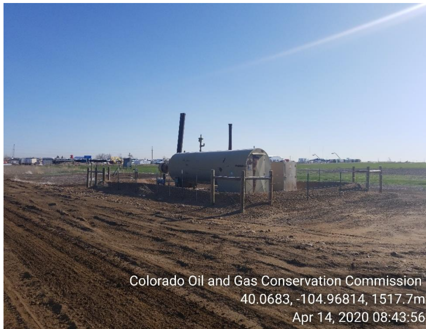
Photo 2 Separators and meter run
