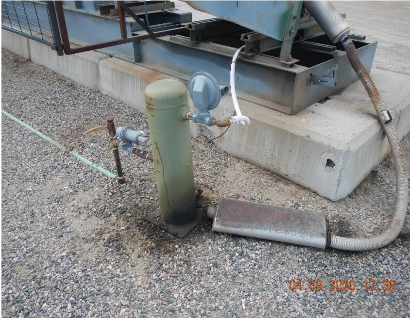
Stained soil at prime mover exhaust for the #4-1.
