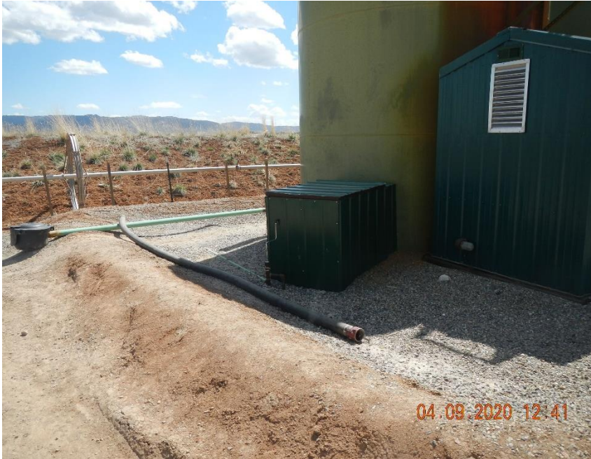
Hose stored in secondary containment for tank battery.
