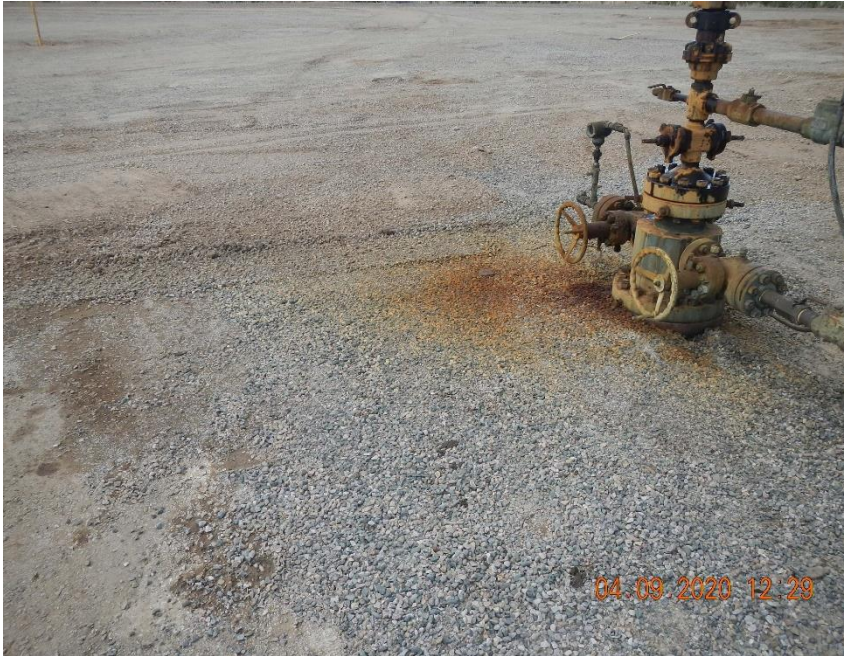
Wet and stained soil and gravel around #4-4 well head.
