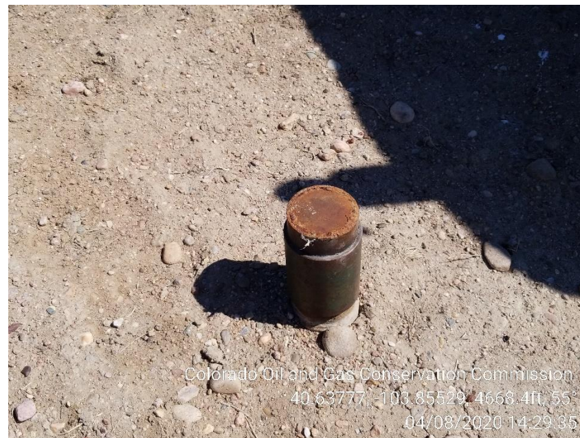
Photo 2 – Well Bore has been covered at Surface
