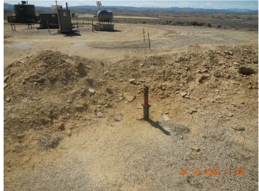
Photo 2. Riser not marked for abandonment or LOTO.
