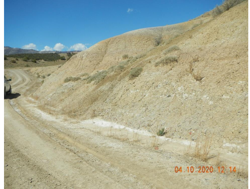
Sediment build up in ditch
