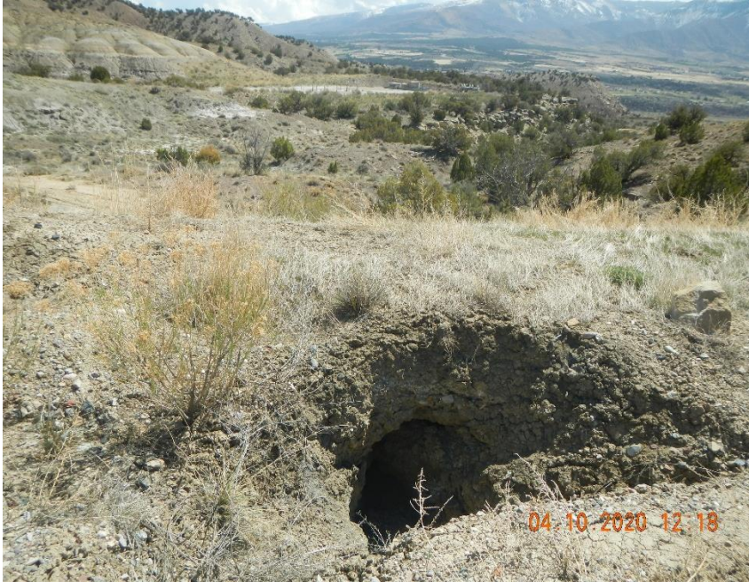
Channeling of road shoulder/berm.
