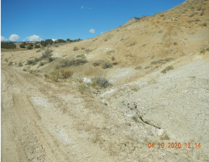
Washing of road at culvert. Lat/Long 39.472689 -108.055189
