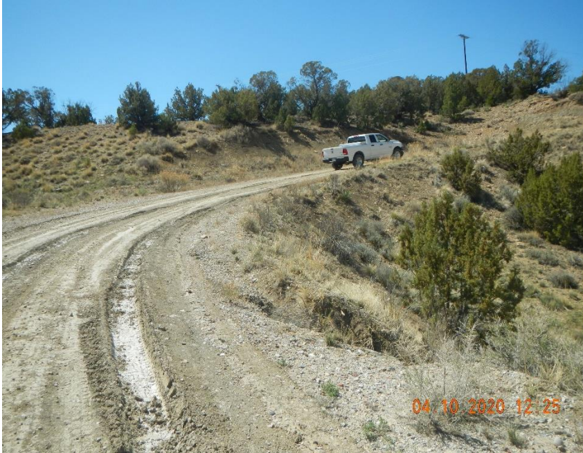
Erosion of road shoulder. Lat/Long 39.472178 -108.056422
