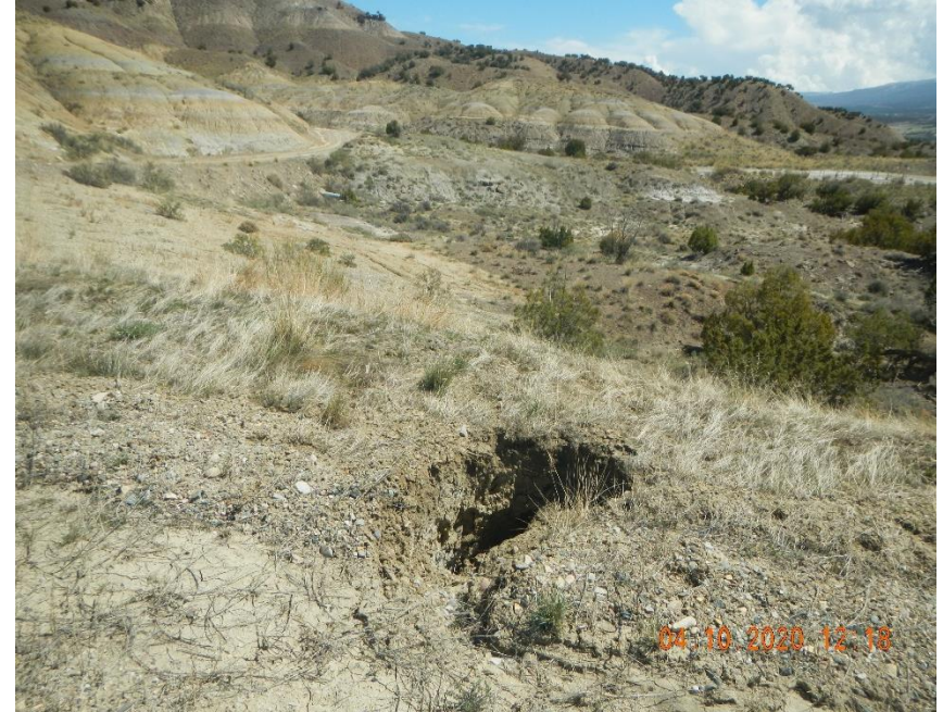
Channeling of road shoulder/berm. Lat/Long 39.472494 108.056294
