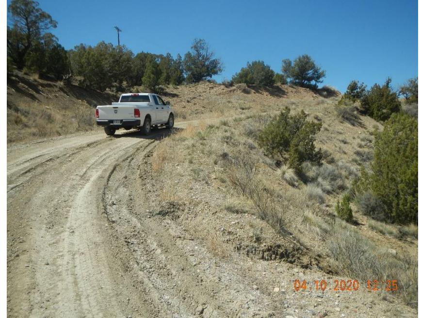
Erosion of road shoulder.
