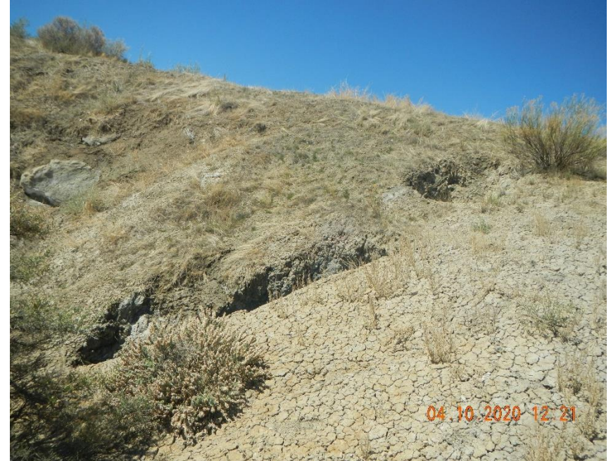
Channeling of road shoulder/berm.
