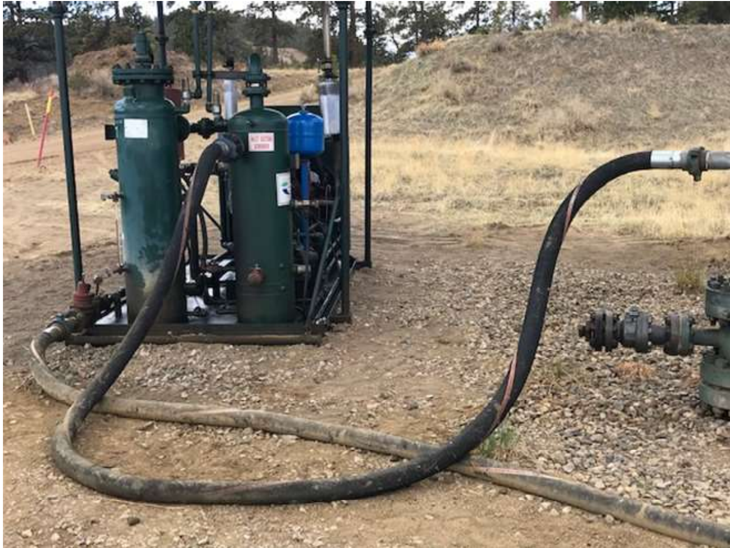
PHOTO 4: THE LEAKS FROM THE LIQUID RING COMPRESSOR WERE IDENTIFIED AND REPAIRED. THE LIQUID RING SKID WAS CLEANED UP ONCE THE REPAIRS WERE COMPLETED.
