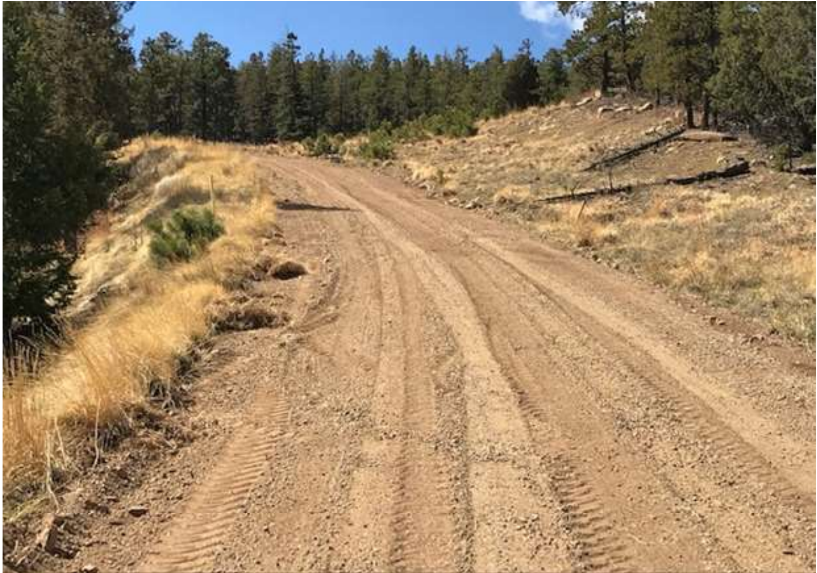
PHOTO 7: THE MAIN LEASE ROAD WAS SURFACED CROWNED TO CREATE SHEET FLOW AND ELIMINATE THE SURFACE EROSION.
