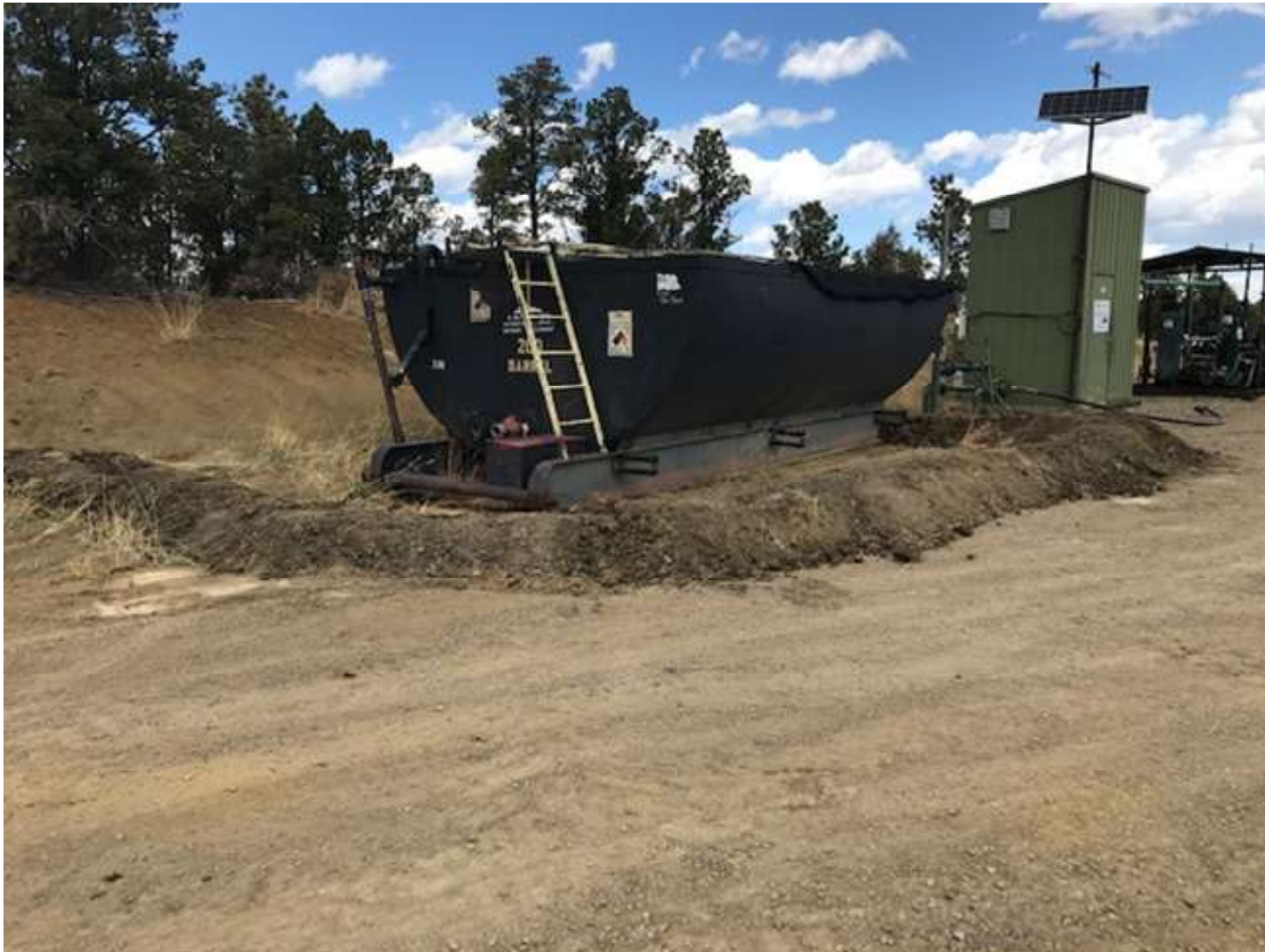
PHOTO 4: A DIRT BERM WAS INSTALLED AROUND THE 200 BBL WATER STORAGE TANK TO PROVIDE SECONDARY CONTAINMENT.
