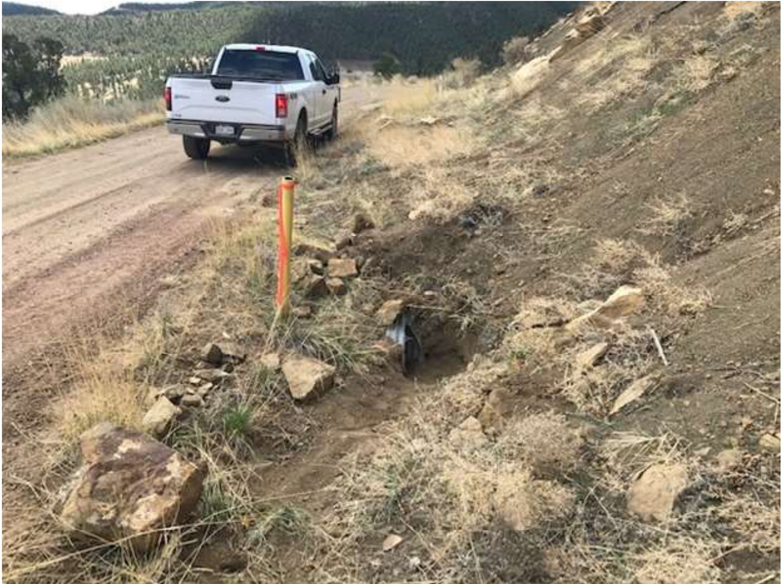
PHOTO 3: THE SEDIMENT ACCUMULATION WAS REMOVED FROM THE CULVERT INLET ALONG THE MAIN LEASE ROAD.
