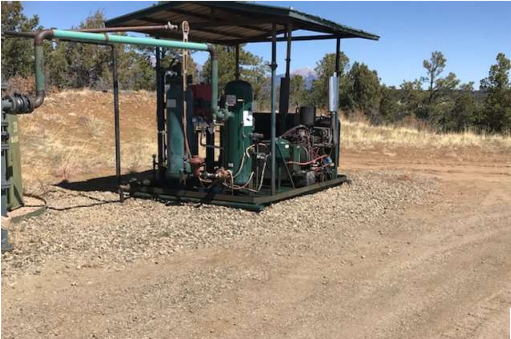
PHOTO 5: THE EXHAUST PIPE EXTENTION WAS USED DURING THE WINTER TO KEEP THE COMPONENTS ON THE LIQUID RING COMPRESSOR FROM FREEZING. THE EXTENTION IS NOT IN USE DURING THE SUMMER AND WAS REMOVED FROM THE LOCATION. THE MUFFLER WAS REPLACED AND IS IN GOOD MECHANICAL CONDITION.
