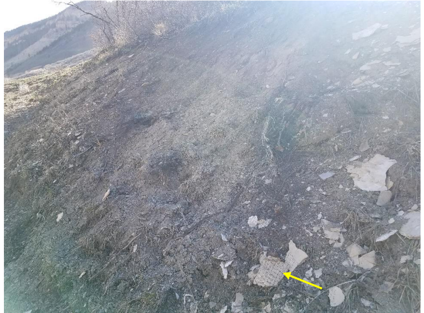
Photo 6: Photo taken from the cut slopes on the southeast end of the Location. Photo shows erosion netting; Netting shows signs of disrepair; Maintenance advised.
