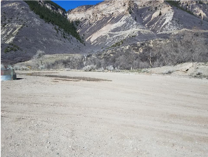
Photo 5: See comments under photo 2. Photo also shows large areas of cut slope that are exposed and at risk of erosion degradation.
