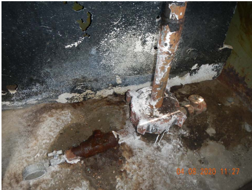
Photo 1. Stained soil at wellhead.
