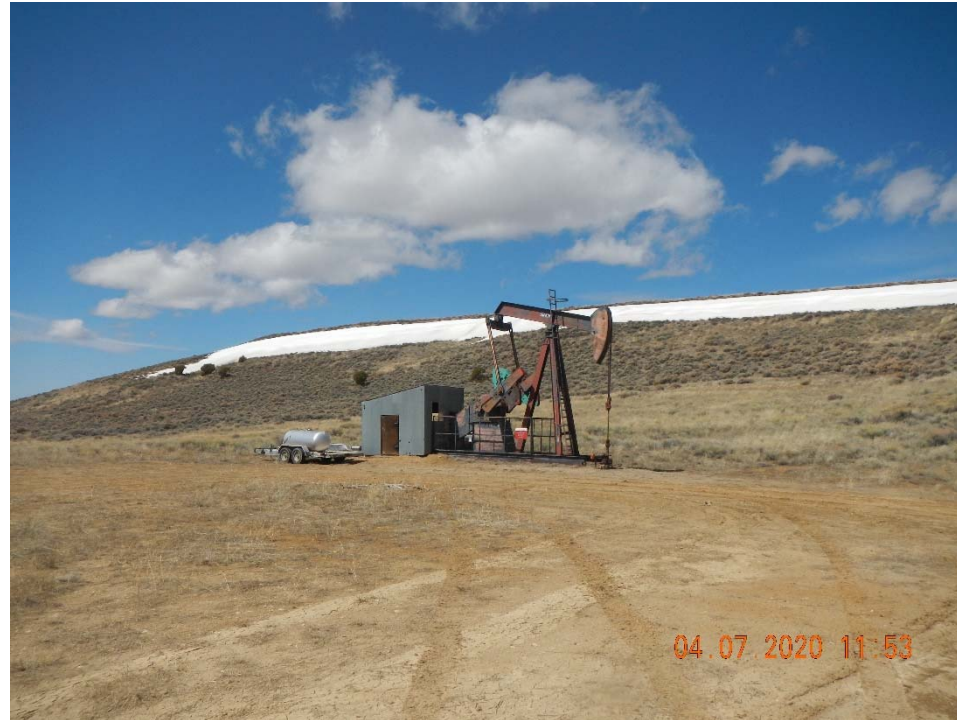
Photo 1. Overview of location taken facing west.
