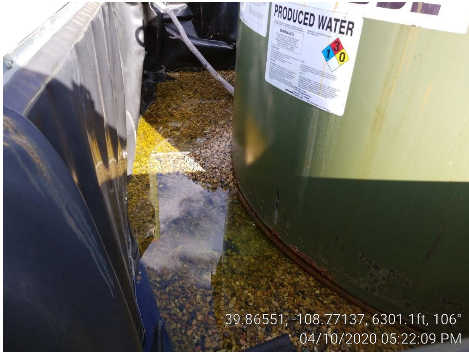
Photo 3. Fluid in secondary containment.
