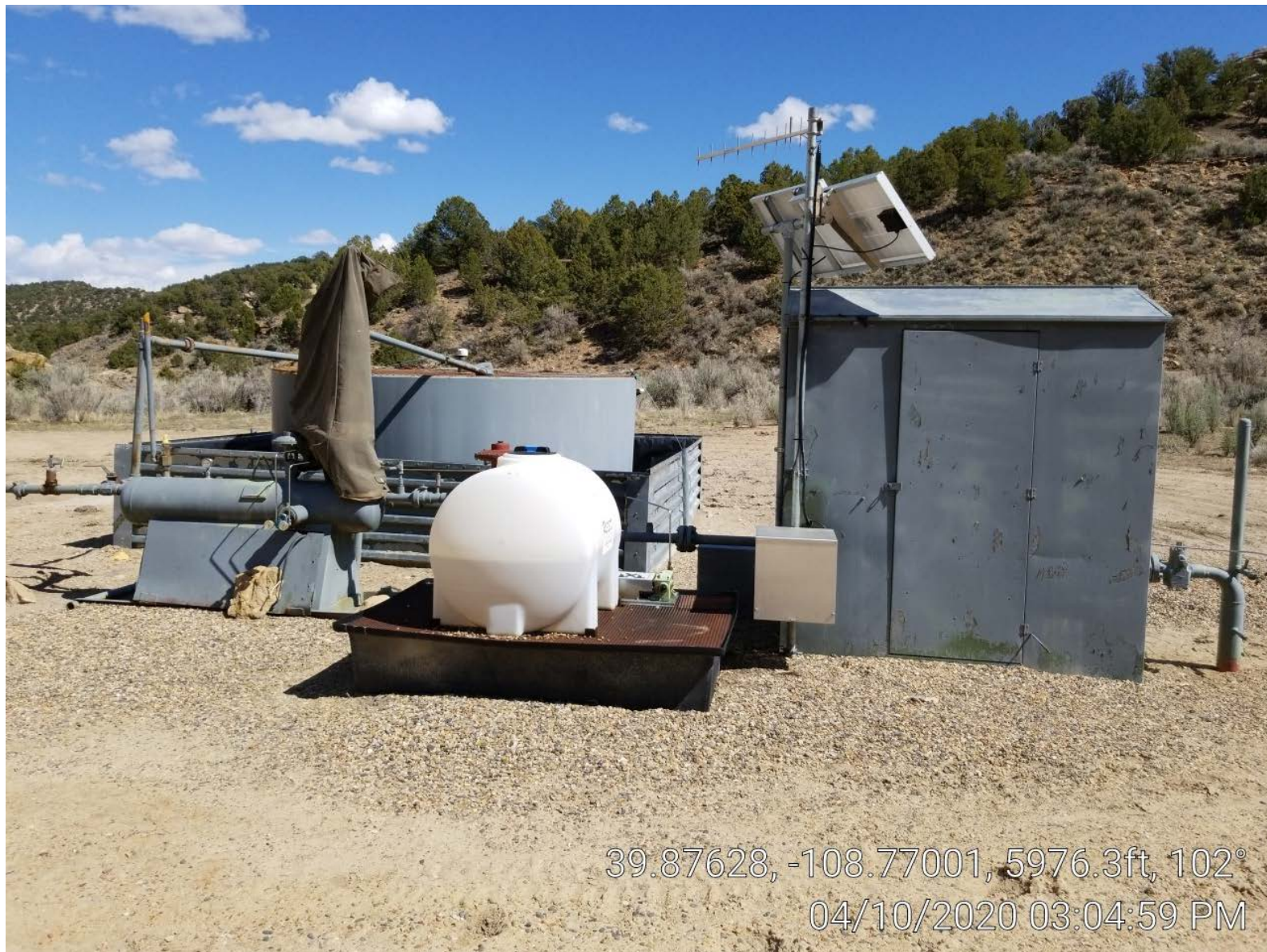
Photo 2. Tank, separator, and meter building.
