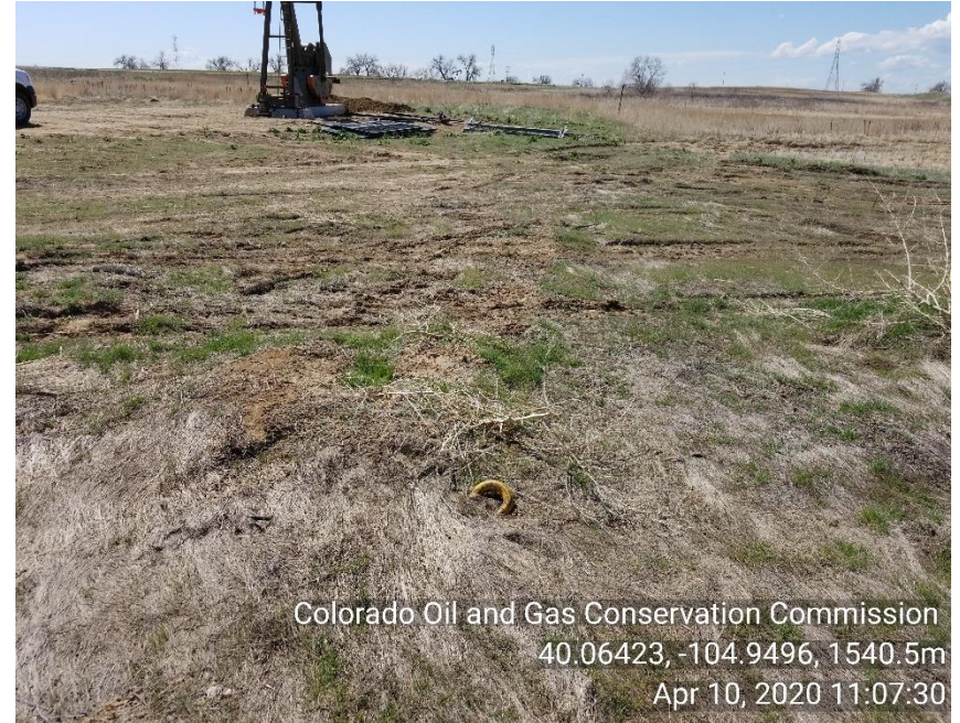
Photo 6 Guyline anchor not properly marked
