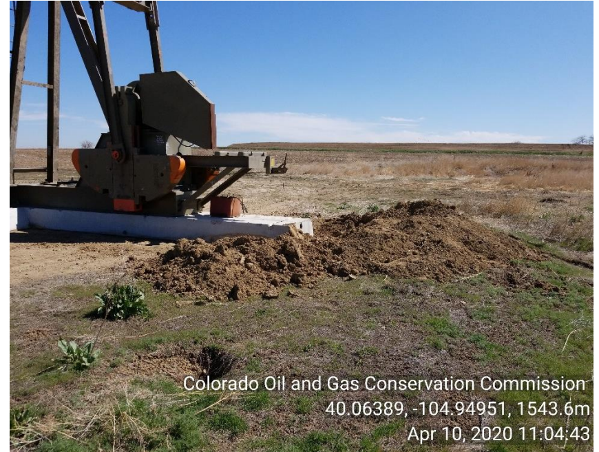
Photo 4 No storm water BMP's in place to protect soils.
