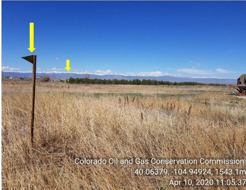
Photo 5 Guy line anchor not properly marked and dead weeds on location.
