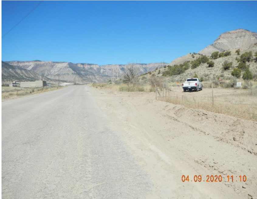
Storm water sediment moving from access roads onto shoulder of county road.
