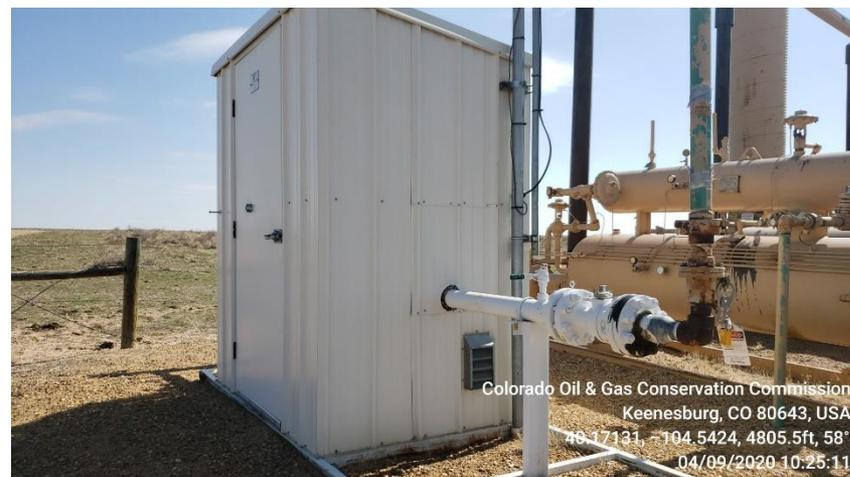
Photo 5 Horizontal Heated Separators
