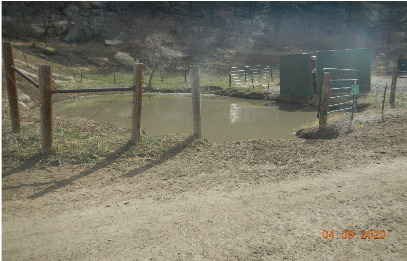
Photo 1. Facing toward the pit at the location. Water level in pit is above freeboard.
