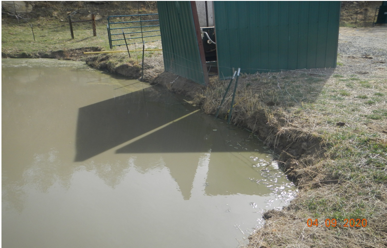
Photo 2. Water level in the pit is above the freeboard marker.
