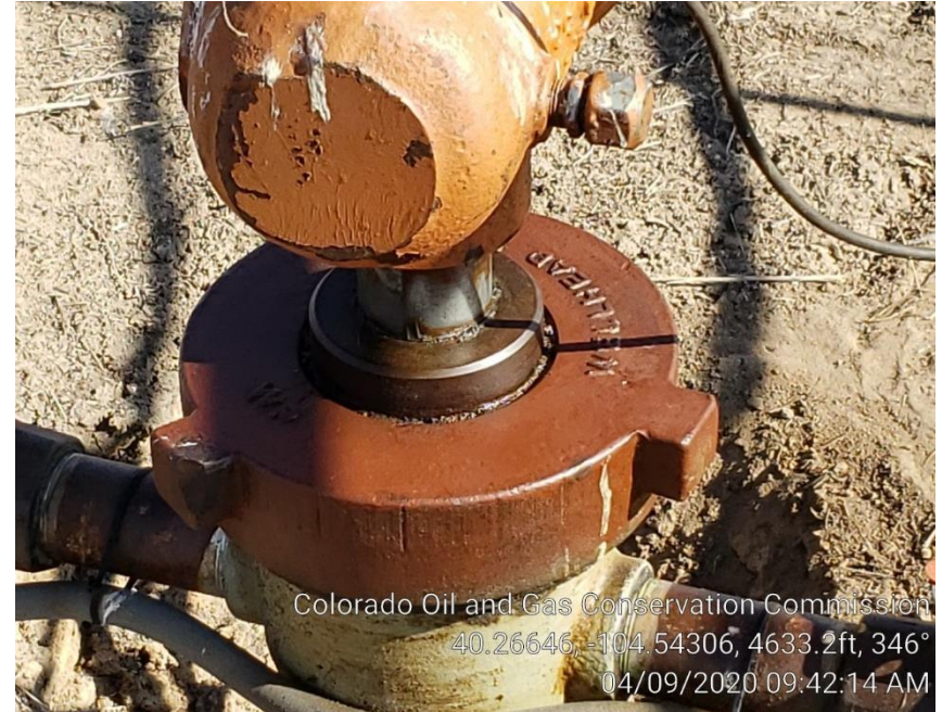
Photo #4 no fluid on surface casing
