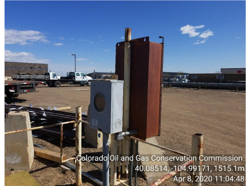
Photo 2 No meter on electric panel and breaker in the off position. Pumping unit is not able to operate with out power.
