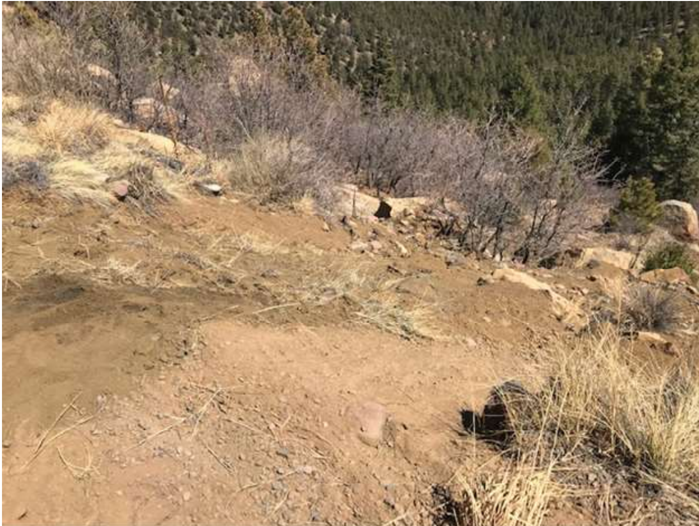
PHOTO 2: THE EROSION ON THE FILL SLOPE WAS ADDRESSED BY BACK FILLING THE DITCH AND THE CPW APPROVED SEED MIX WAS HAND BROADCAST TO PROMOTE THE ESTABLISHMENT OF VEGETATION.
