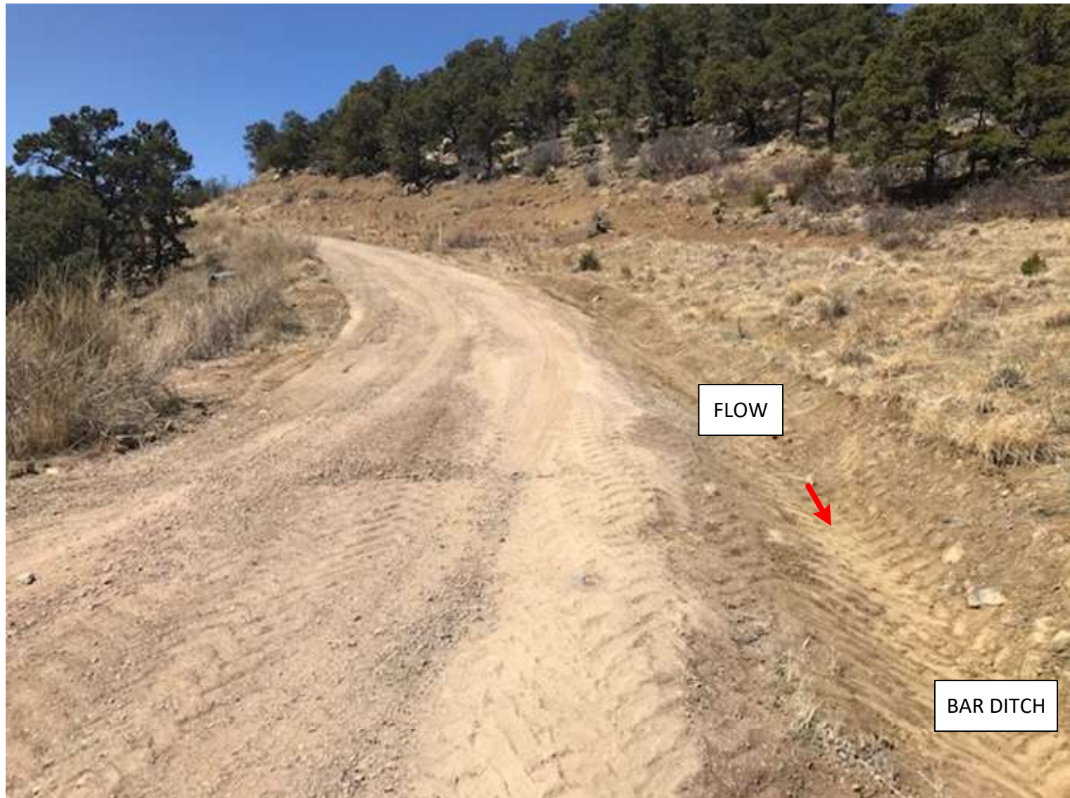
PHOTO 4: THE ACCESS ROAD WAS SURFACE CROWNED TO ESTABLISH SHEET FLOW AND ELIMINATE THE SURFACE EROSION OF THE ACCESS ROAD. THE BAR DITCH WAS DOMINATED TO REDIRECT STORMWATER TO THE DOWN GRADIENT CULVERT INLET.
