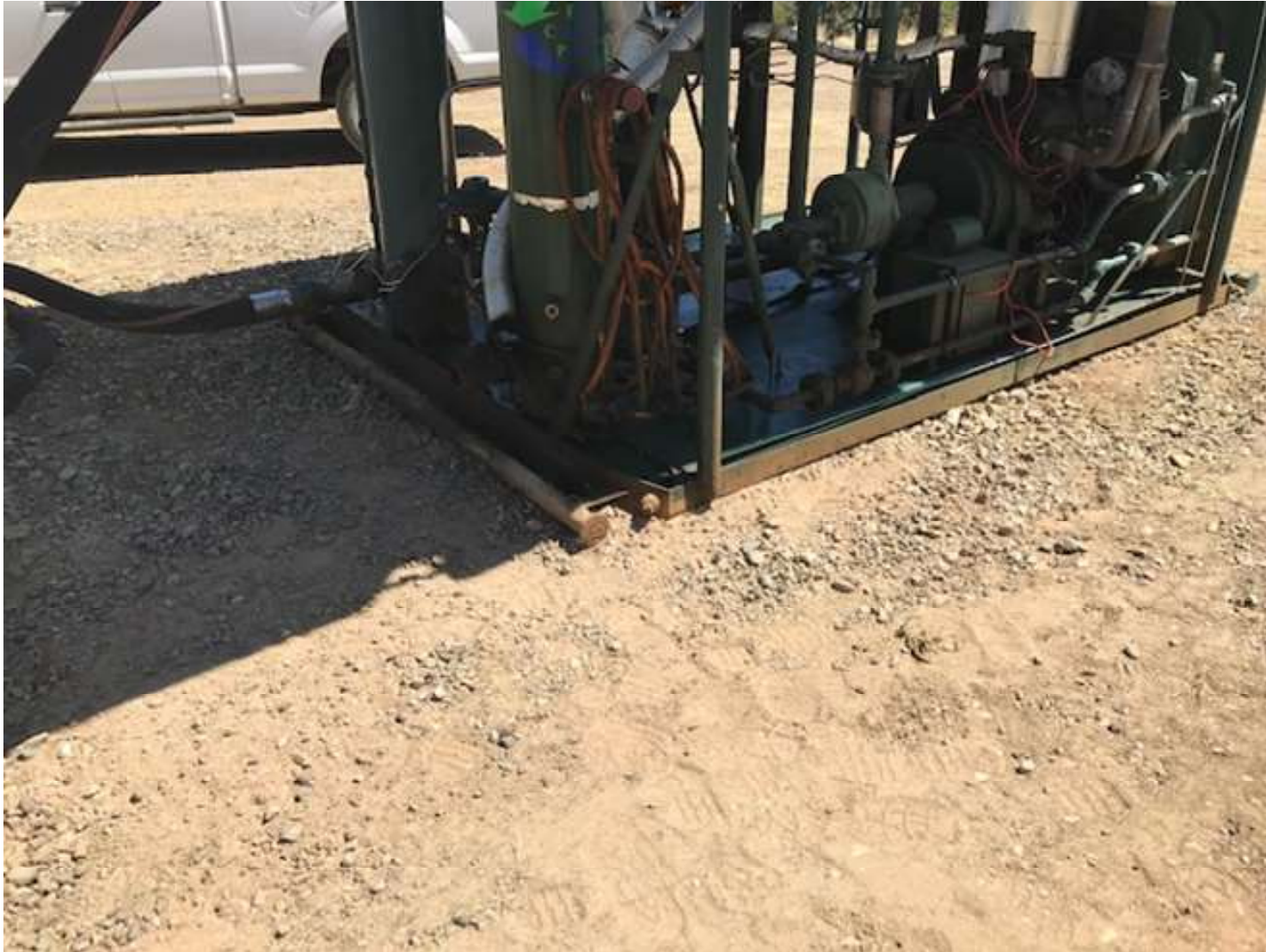
PHOTO 6: THE LIQUID RING SKID AND RESERVIOR HAS BEEN CLEANED AND THE ACCUMULATED FLUID WAS REMOVED. THE IMPACTED SOIL WAS ALSO REMOVED FROM LOCATION.
