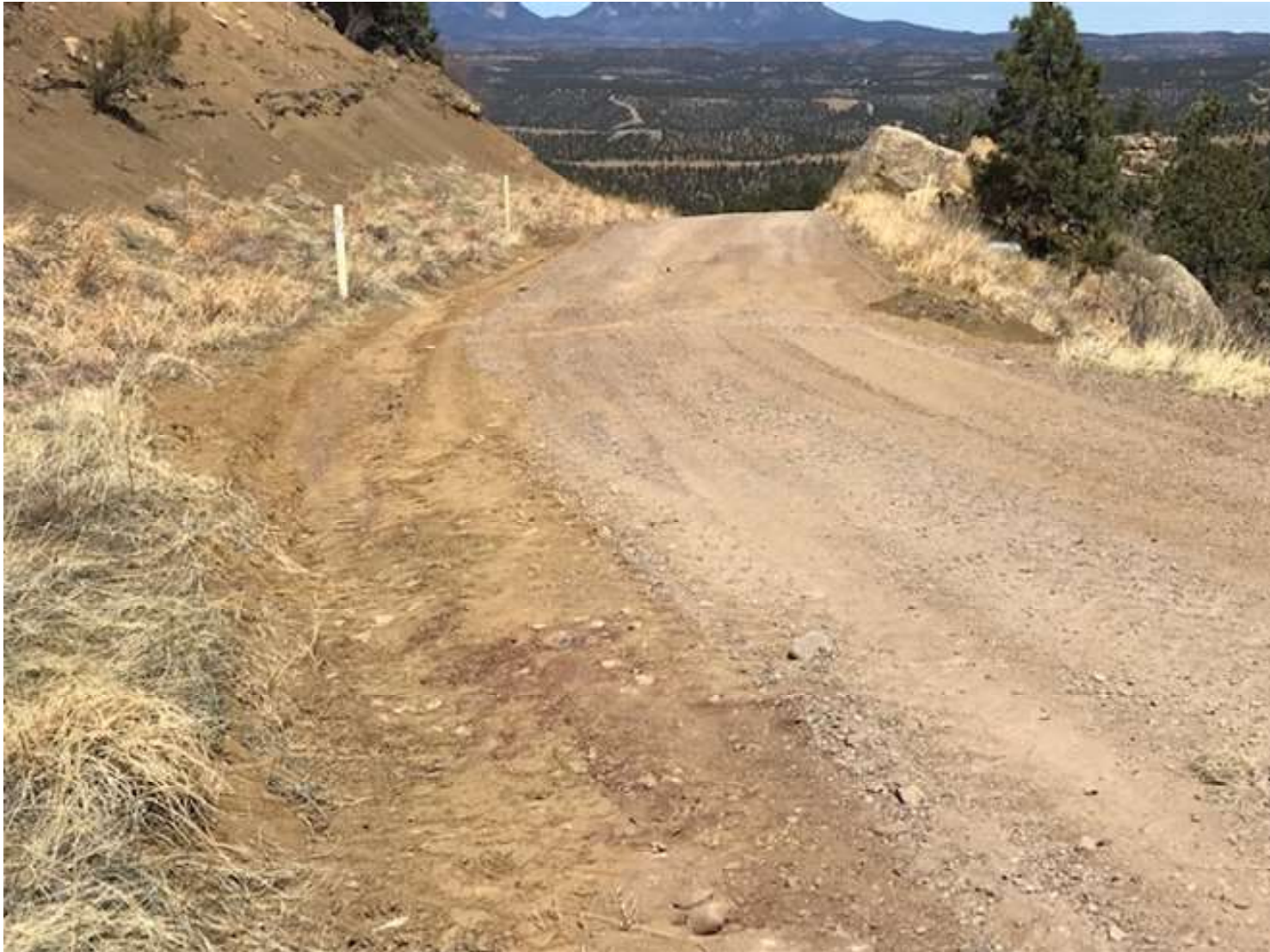
PHOTO 1: THE BAR DITCH PARALLEL TO THE ACCESS ROAD WAS DOMINATED TO REDIRECT STORMWATER TOWARD THE DOWN GRADIENT CULVERT INLET. THE ACCESS ROAD WAS SURFACE CROWNED TO ESTABLISH SHEET FLOW AND ELIMINATE THE SURFACE EROSION OF THE ACCESS ROAD.
