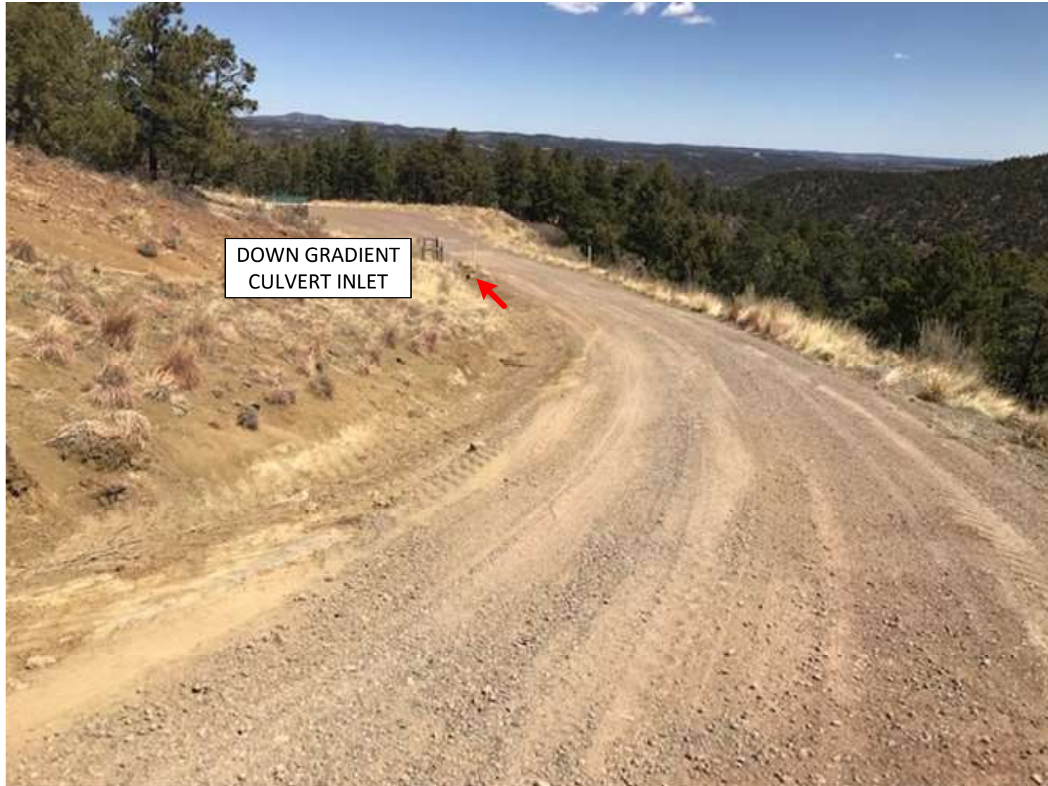
PHOTO 5: THE ACCESS ROAD WAS SURFACE CROWNED TO ESTABLISH SHEET FLOW AND ELIMINATE THE SURFACE EROSION OF THE ACCESS ROAD. THE BAR DITCH WAS RECONFIGURED TO ELIMINATE EROSION.
