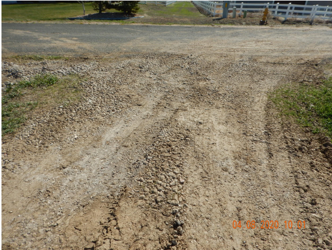
Photo 2. Photo taken from the entrance of location, facing East. Photo illustrates the vehicle tracking device BMP is not in proper functioning condition. Sediment discharge from vehicle tracking was observed on Lansing Ct.
