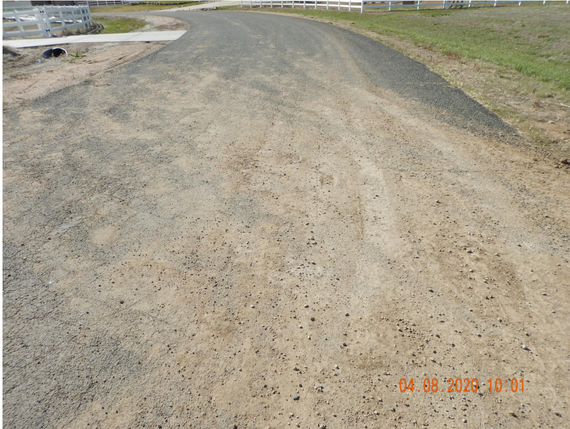
Photo 3. Photo taken from the entrance of location, facing South along Lansing Ct. Photo illustrates sediment discharge from vehicle tracking on Lansing Ct.
