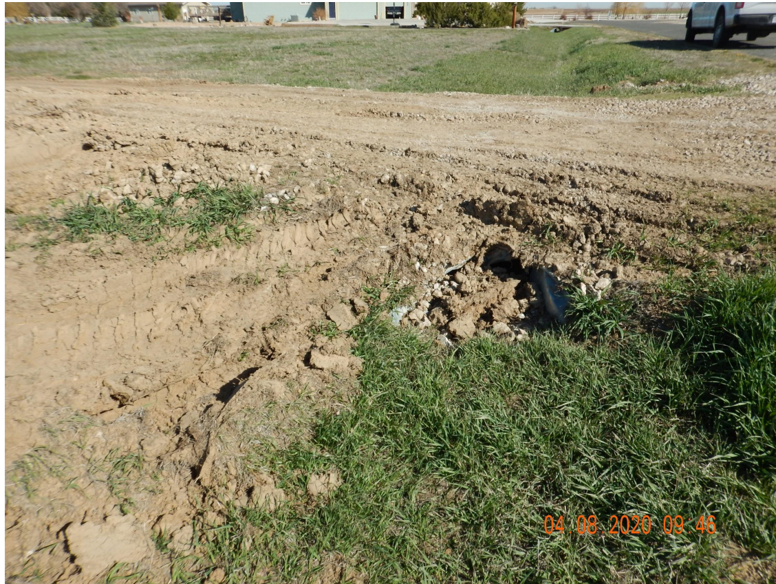
Photo 4. Photo taken from the entrance of location, facing North. Photo illustrates a damaged culvert from vehicle traffic.
