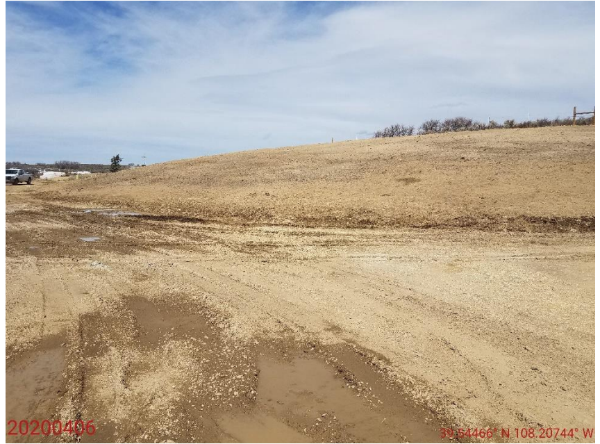
Photo 2: Photo taken from the eastern end of the Location, facing north. Photo shows recent reclamation activities appear to have been conducted on the Location; soils appear to have been recently replaced, contoured, and slopes have been stabilized with a hydromulch.
