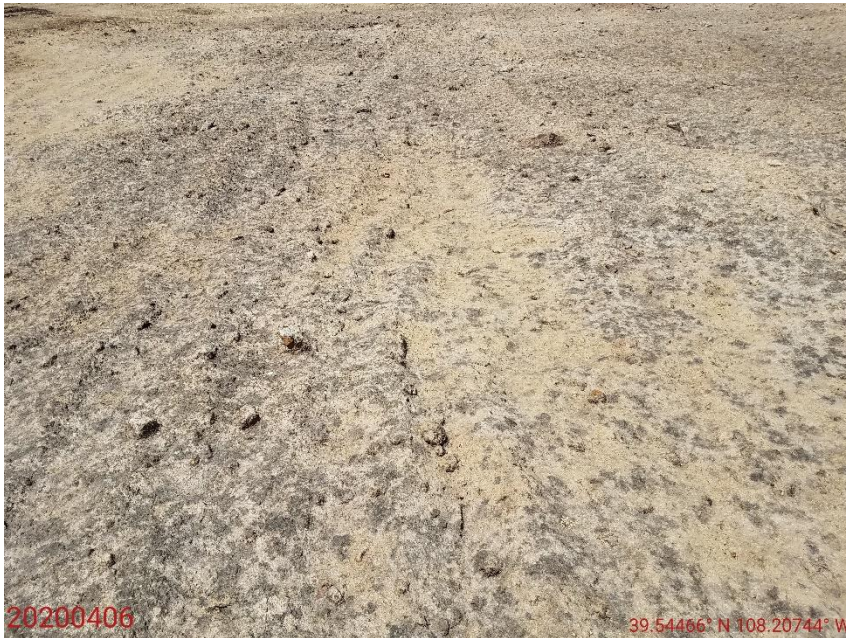
Photo 3: Continued from photo 2. Photo shows hydromulch appears to have been applied to the slopes of the Location, and the interim areas.
