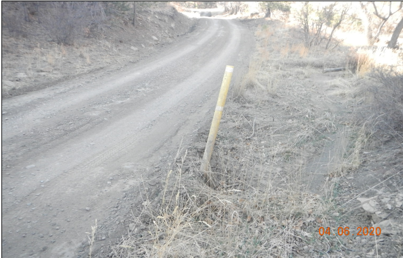
Photo 1. Facing southeast through Little Bingham Canyon. The culvert has filled in with sediment.
