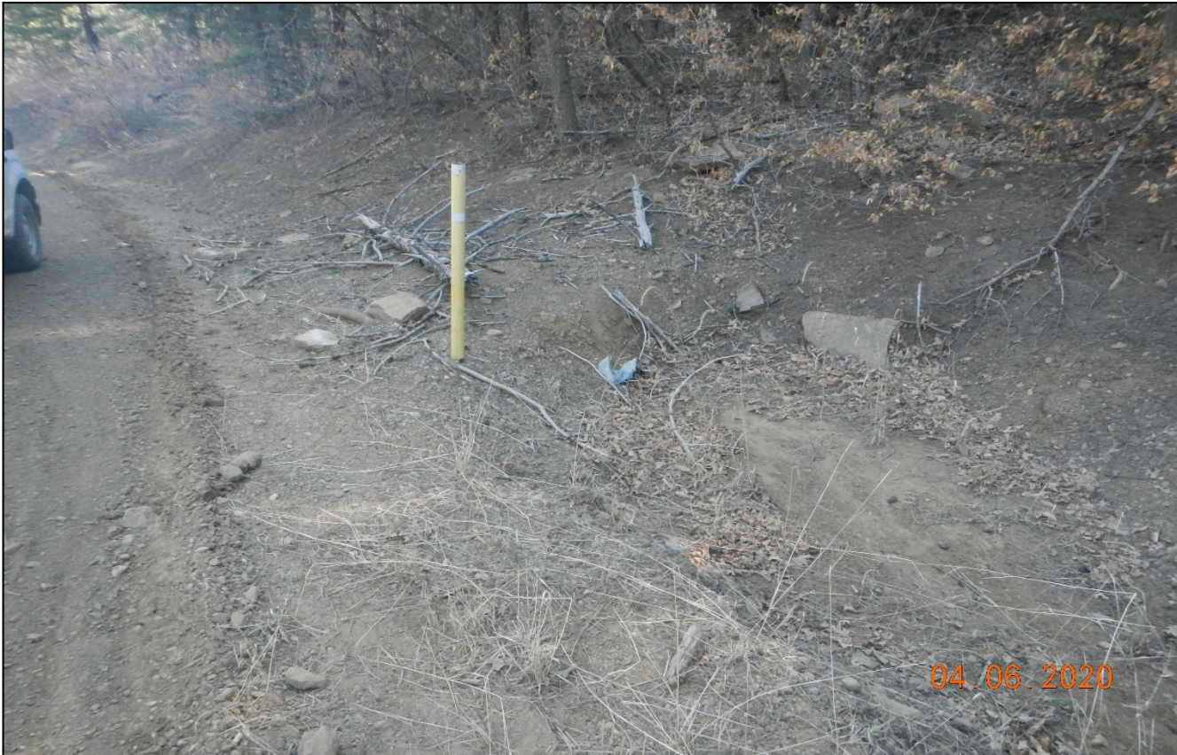
Photo 3. A culvert is filled in with sediment as the road ascends the hill toward the location.
