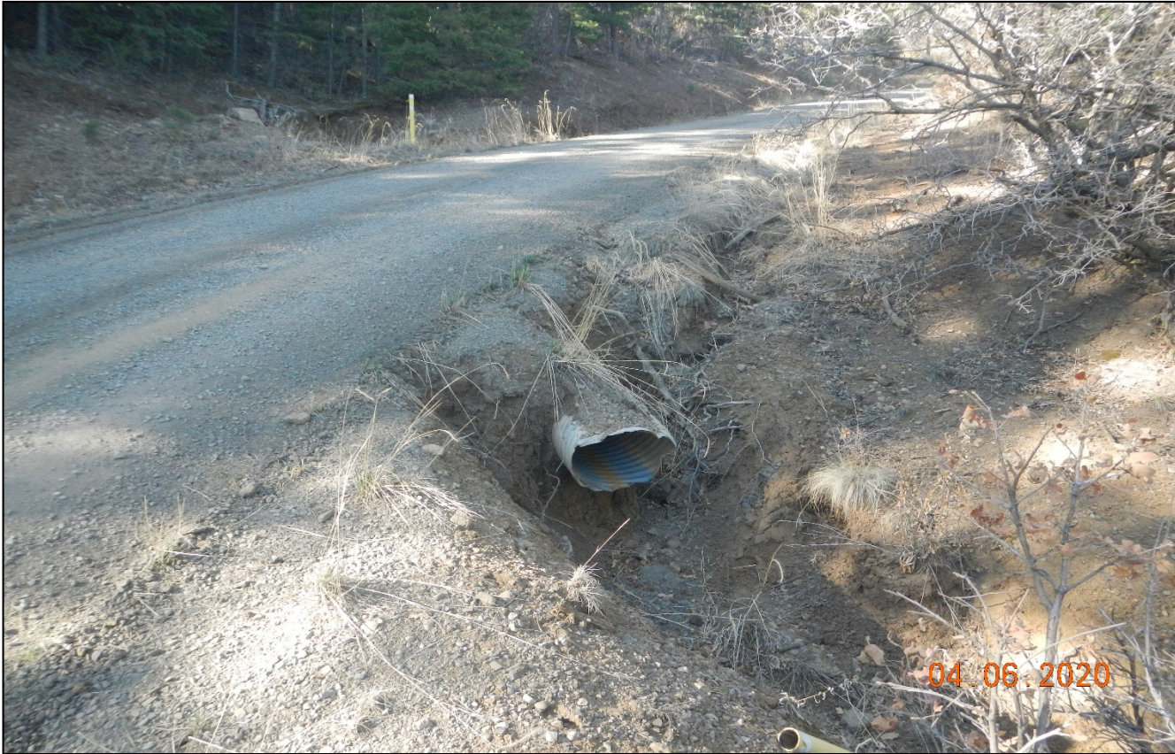
Photo 4. There is erosion occurring at the culvert outlet as the lease road ascends the hill toward the location.
